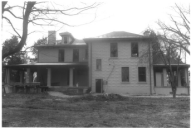
HAYNES HOUSE FRANKLIN CO. TN
