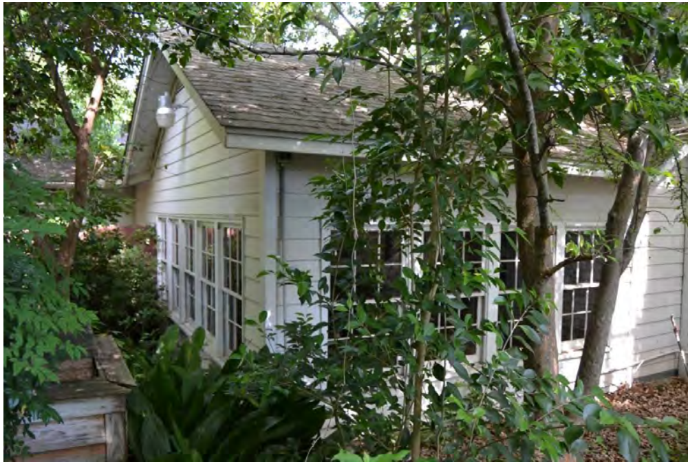
Photo 31. Current photograph (facing southeast) of the dining room extension built sometime after 1985 to the south of the ca. 1960 addition. The design of the additions built after 1985 are compatible with the original 1860 building and allow it to retain sufficient integrity to convey its significance. Source: HHM, 2016.
