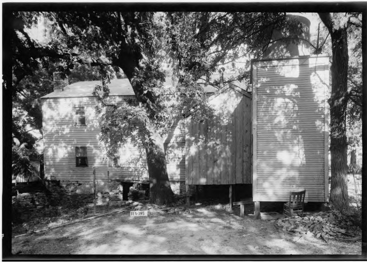
Figure 10. Historic photograph (facing east) from 1936 of the Stagecoach Inn's west (rear) side showing a non-extant rear board-and-batten kitchen addition with a raised water tank. Note the bur oak at center is the tree in the central atrium today. An addition blocks this view currently but Photo 28 partially shows this façade from the atrium. Source: Shady Villa HABS TX-395.
