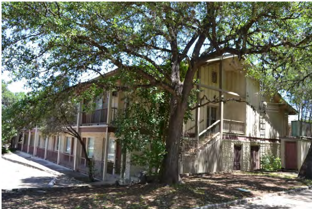
Figure 49. Current photograph (facing northeast) of the 1960 lodging building (Resource 7) at the southwest corner of the property. Note the board-and-batten siding, painted brick with squeezed mortar joints, and the exposed post-and-beam feature surrounding the exterior stairwell. Unlike the other original lodging buildings (Resources 5 and 6), this building is two-rooms deep with an interior central hallway. Source: HHM, 2016.
