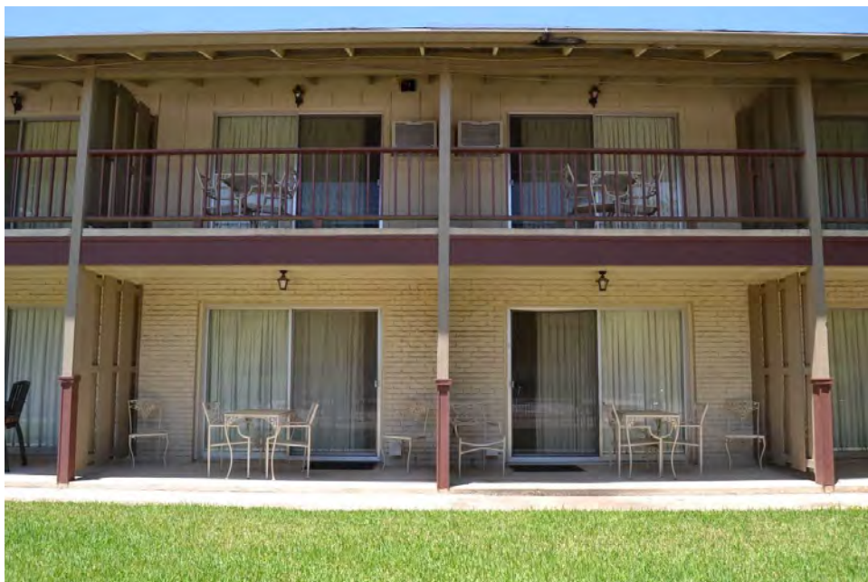
Photo 47. Current photograph (facing north) of the 1960 lodging building (Resource 5) north of the central pool area. Note the board-and-batten siding, painted brick with squeezed mortar joints and original wrought iron patio furniture. Source: HHM, 2016.
