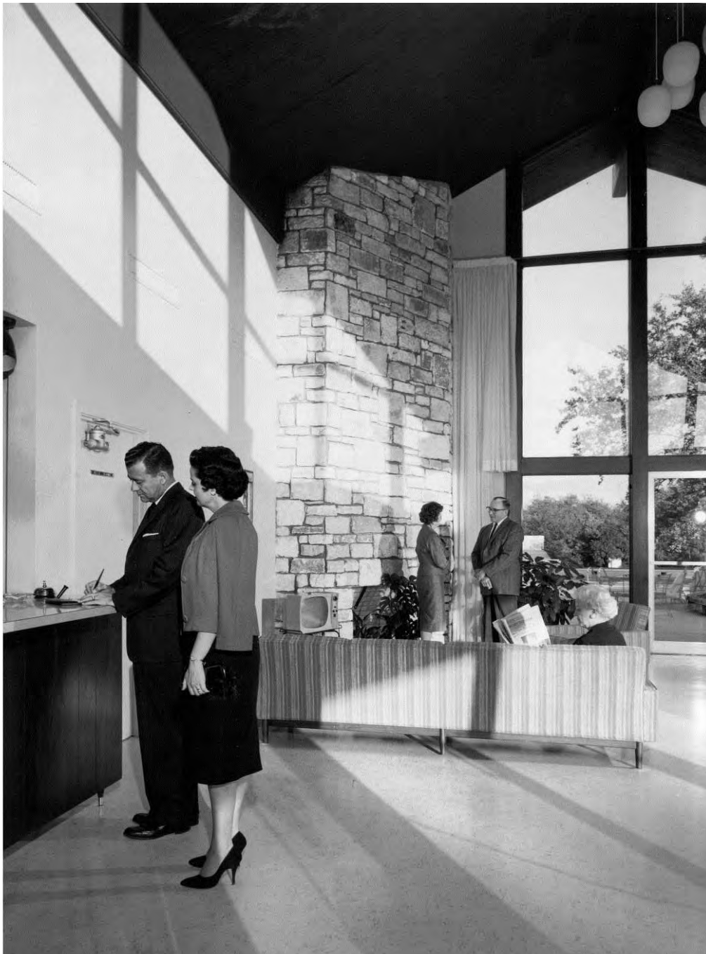
Figure 19. Historic photograph (facing east) from 1960 of the interior of the lobby building (Resource 3). The flooring, lighting fixtures, and furniture have been replaced. Compare with the current photograph in Photo 37. Source: Stagecoach Inn archives, Salado, Texas.
