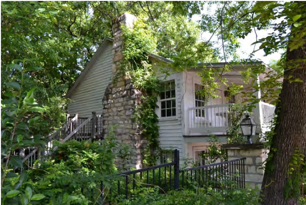
Photo 14. Current photograph (facing northwest) of the east (front) and south sides of the 1860 building. A second external chimney to the rear of the current stone chimney was removed in the 1940s. The wood stairway to the left is not original. Compare to the historic photographs in Figures 5 and 11. Source: HHM, 2016.
