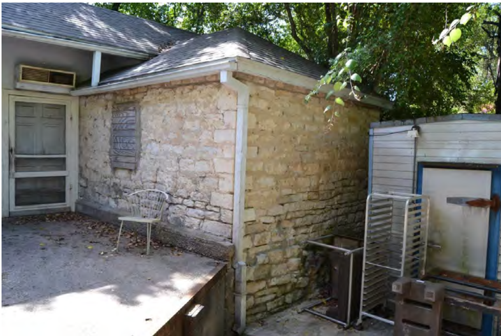
Photo 23. Current photograph (facing southeast) of the pre-1936 stone smokehouse. Once a freestanding outbuilding, the smokehouse was incorporated into later rear additions to the inn and is now used for kitchen storage. Compare to the historic photograph in Figure 12. Source: HHM, 2016.
