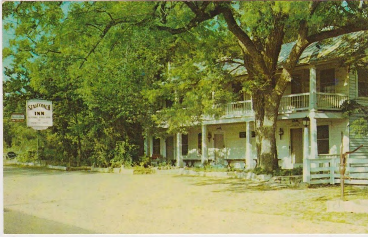
Figure 15. Historic photograph (facing southwest), possibly from the late 1940s or 1950s of the front of the Stagecoach Inn. Note the sign which reads "Stagecoach Inn, Historical Stage Stop of Pioneer Days," the spring water well (non-extant) to the right, and the misaligned ground floor columns, a post-1935 modification that was restored to regular spacing after 1981. Compare with the current photograph in Photo 12. Source: Postcard sold on eBay, link not available.
