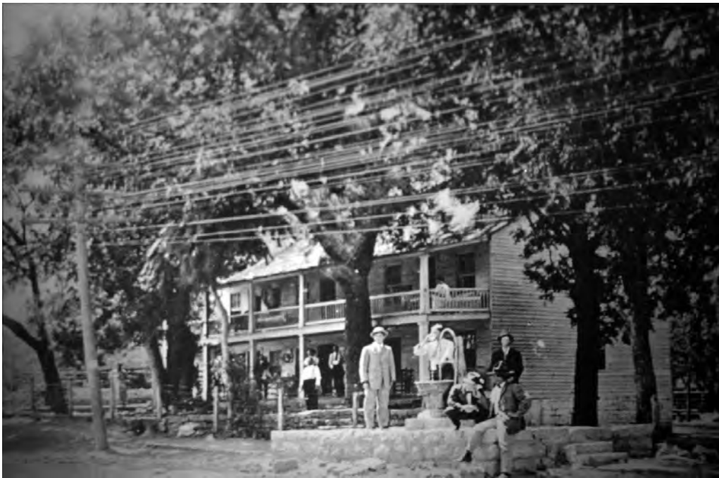
Figure 4. Historic photograph (facing southwest), possibly from the mid-1930s of the front of the Stagecoach Inn and the street-side spring water well when newspapers documented the construction of a new well. Compare with the current photograph in Photo 12. Source: Hodge.
