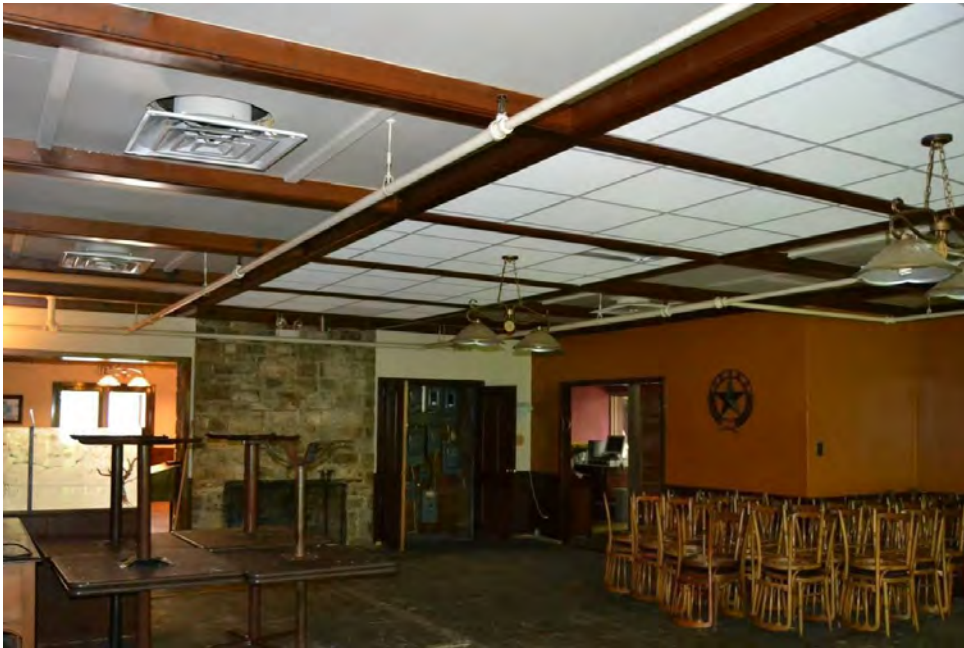
Photo 26. Current photograph (facing east) of the 1960 dining room addition to the rear of the original 1860 building. The stone fireplace and wood ceiling coffers are original. All other finishes and fixtures have been replaced. Compare to the historic photograph in Figure 23. Source: HHM, 2016.
