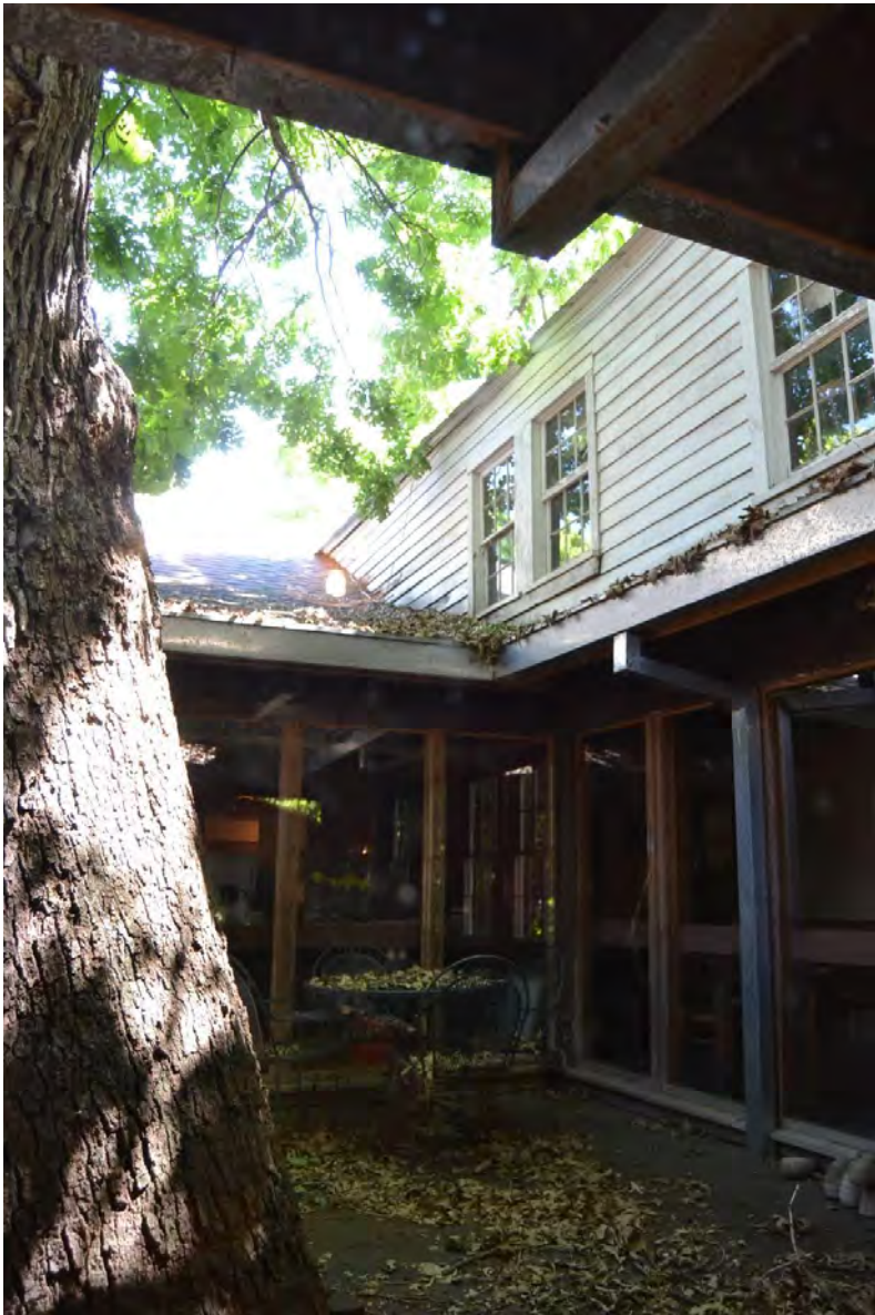
Photo 28. Current photograph (facing north) of the west (rear) side of the 1860 building (visible with horizontal wood siding) and its ca. 1960 rear addition surrounding a large bur oak, taken from the central atrium. The double windows on the upper floor may be original but are not in their original configuration. Compare to the historic photograph in Figure 10. Source: HHM, 2016.
