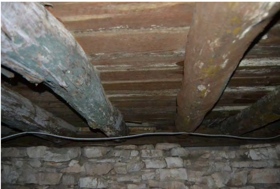
Photo 21. Current photograph (facing east) of the crawl space under the first floor of the original 1860 building showing un-hewn logs used as floor joists. In many locations throughout the building, un-hewn and rough-hewn wood structural elements are visible. Source: HHM, 2016.
