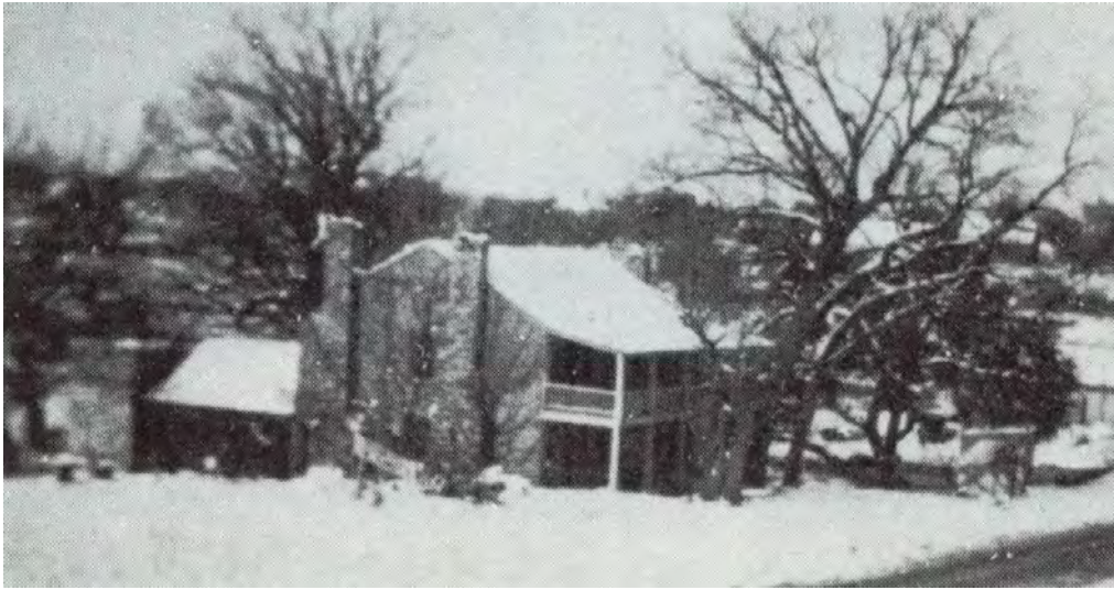
Figure 5. Historic photograph (facing north) after a snow storm of the Stagecoach Inn's south side in the early-to-mid 1930s, clearly showing both end chimneys and a non-extant rear kitchen addition with a raised water tank. Figure 10 shows these past rear additions more clearly. Compare with the current photograph in Photo 14. Source: Cutler.
