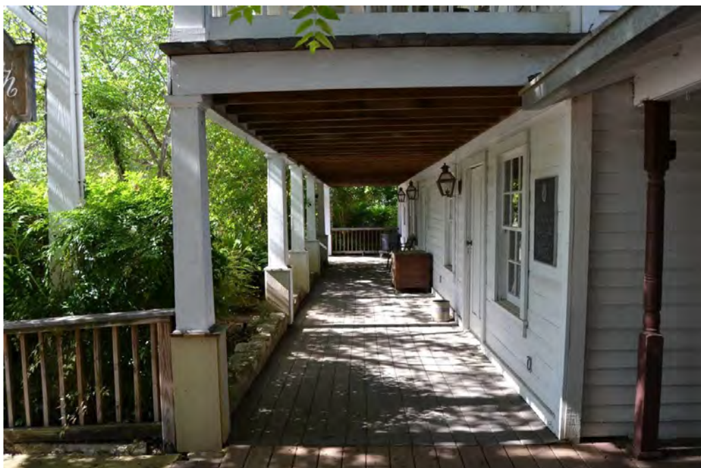
Photo 13. Current photograph (facing south) of the front porch of the 1860 building. The porch floor and the bases of the porch columns have been replaced. Compare to the historic photograph in Figure 26. Source: HHM, 2016.
