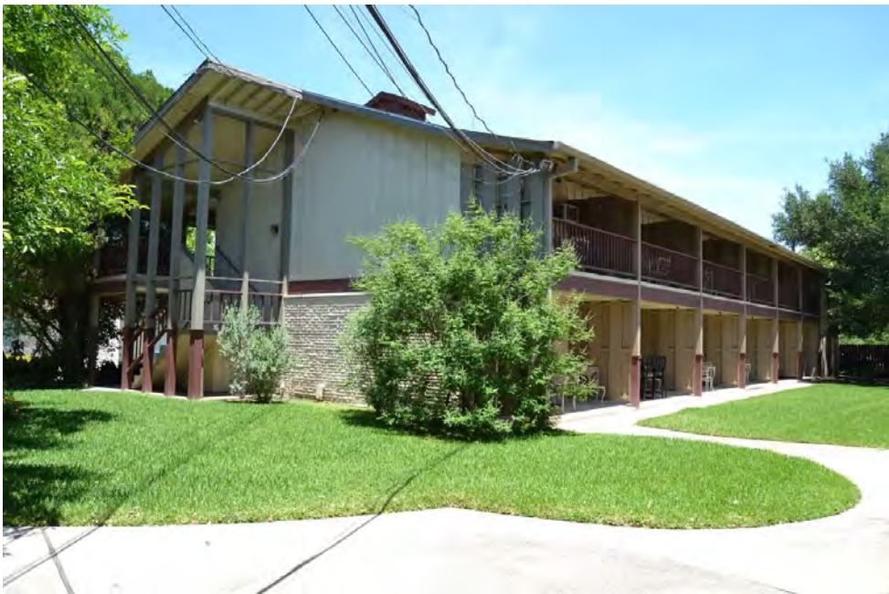
Photo 45. Current photograph (facing northeast) of the 1960 lodging building (Resource 5) north of the central pool area. Note the board-and-batten siding, painted brick with squeezed mortar joints, and the exposed post-and-beam feature surrounding the exterior stairwell. This building is one-room deep with room entrances on both sides of the building. Source: HHM, 2016.
