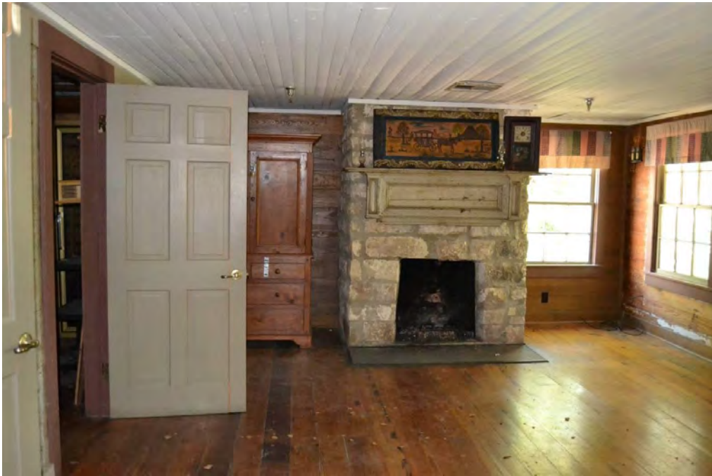
Photo 18. Current photograph (facing north) of the northeastern fireplace on the second floor of the original 1860 building. Fireplace details and hardware have changed. Wooden floors, walls, ceilings, and window and door trim likely date to the period of significance. Source: HHM, 2016.
