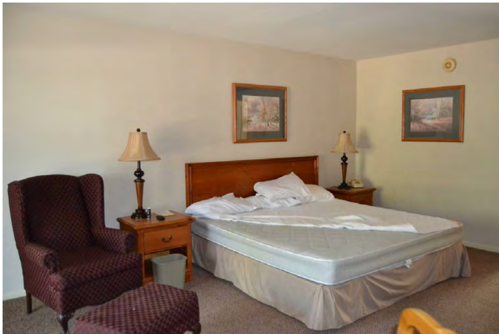
Photo 48. Current photograph at typical room in the 1960 lodging building. All fixtures, finishes and furniture have been replaced. Compare with historic photograph in Figure 22. Source: HHM, 2016.
