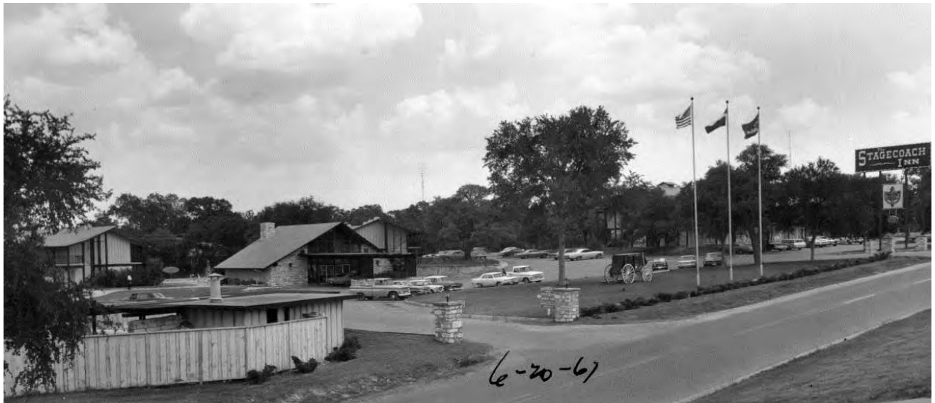
Figure 24. Historic photograph (facing southeast) dated June 20, 1961, of the Stagecoach Inn motel resort entrance, from the I-35 frontage road. Visible is the lobby building (foreground, Resource 3) and the three surrounding lodging buildings (Resources 5, 6, 7). Compare with the current photograph in Photo 2. Source: Stagecoach Inn archives, Salado, Texas.
