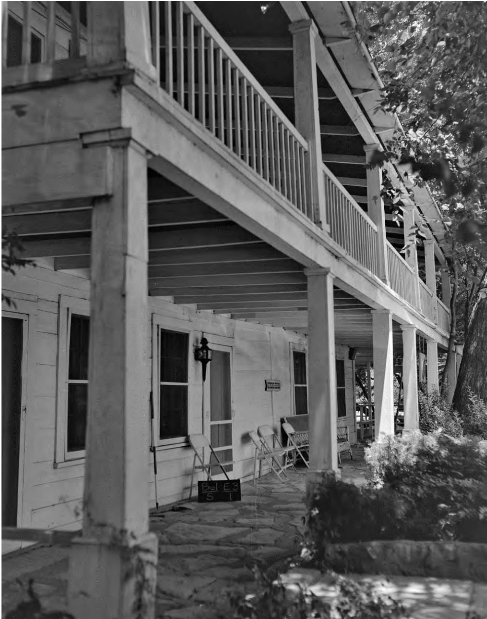
Figure 26. Historic photograph (facing north) from 1970 of the front porch of the Stagecoach Inn. The stone porch floor has been replaced with composite wood boards, the window and door screens have been removed, and the light fixtures have been replaced. Compare with the current photograph in Photo 13. Source: The Portal to Texas History, University of North Texas Libraries, crediting Texas Historical Commission, https://texashistory.unt.edu/ark:/67531/metaph680516/ , accessed October 17, 2016.
