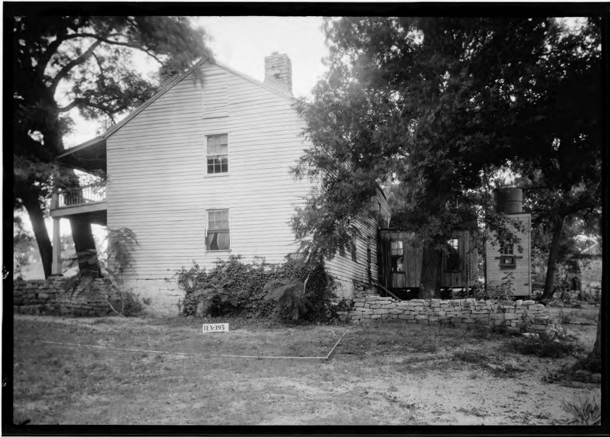
Figure 9. Historic photograph (facing south) from 1936 of the Stagecoach Inn's north side, showing both internal chimneys at this end (rear chimney is not extant) and a non-extant rear board-and-batten kitchen addition with a raised water tank. Note the bur oak directly in front of the rear kitchen is the tree in the central atrium today. The window configuration on this façade has been altered. An addition blocks this view currently but Photo 12 partially shows this façade. Source: Shady Villa HABS TX-395.
