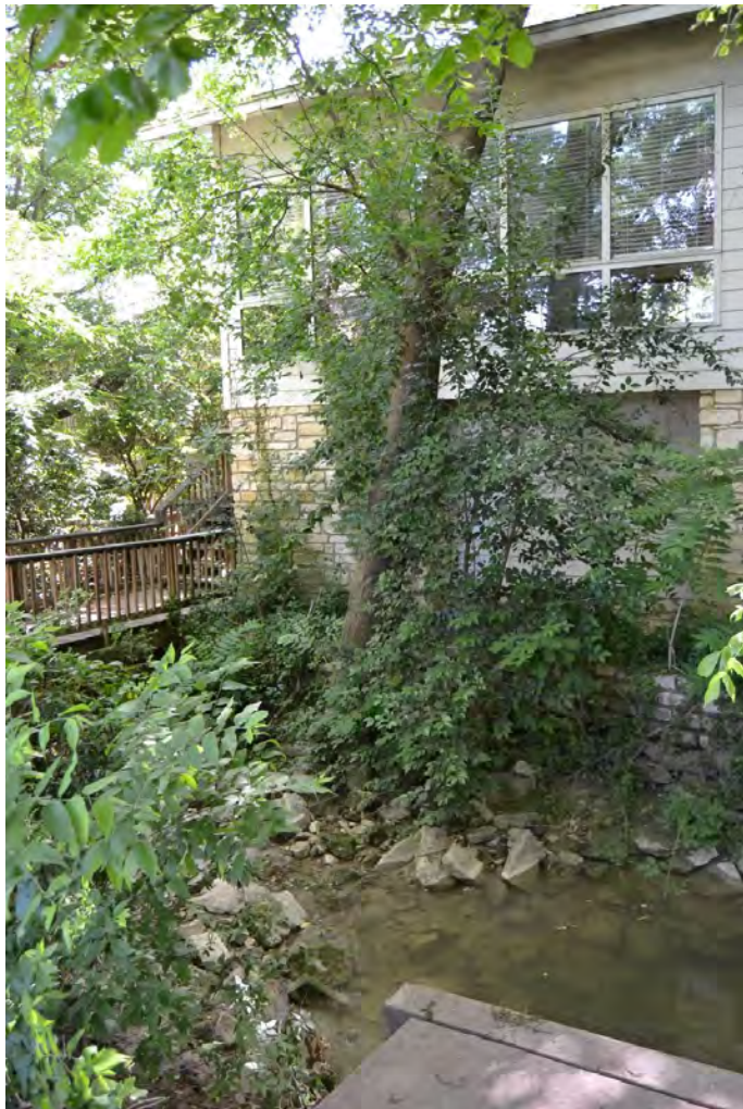
Photo 5. Current photograph (facing east) of the northwest corner of the restaurant (Resource 1), showing the post-1985 addition next to the small stream running through the property. Source: HHM, 2016.
