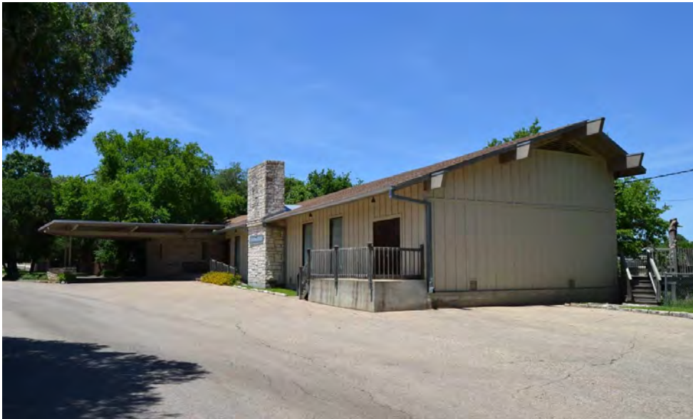
Photo 44. Current photograph (facing west) at the east side of the 1960 clubhouse building (Resource 4), showing the ca. 2005 addition to the building (including the chimney). The design of the addition is compatible with the original 1960 building and allows it to retain sufficient integrity to convey its significance. Source: HHM, 2016.
