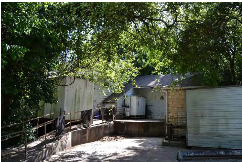
Photo 30. Current photograph (facing east) of the inn's rear additions. The stone structure is an original pre-1936 smokehouse. The other structures are a combination of additions constructed in phases after 1943. Compare to the historic photographs in Figures 12 and 30. Source: HHM, 2016.
