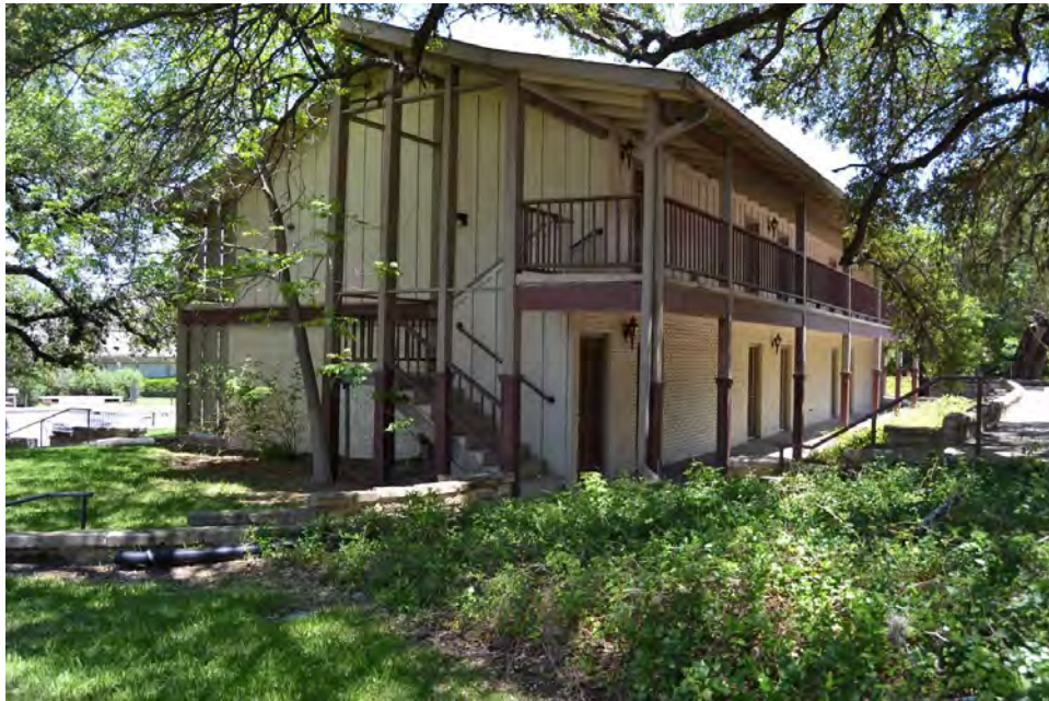
Photo 46. Current photograph (facing northeast) of the 1960 lodging building (Resource 6) south of the central pool area. Note the board-and-batten siding, painted brick with squeezed mortar joints, and the exposed post-and-beam feature surrounding the exterior stairwell. This building is one-room deep with room entrances on both sides of the building. Source: HHM, 2016.
