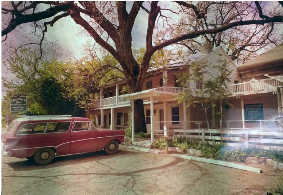
Figure 25. Historic photograph (facing southwest) April 1963, showing the front of the old inn and part of its 1960 rear addition, including a non-extant covered walkway. The roof edge seen at the very right is part of the adjacent log cabin. The large pecan tree at center was removed after 1981. Compare with Photo 12. Source: Texas Department of Transportation, Communications Division, Media Production, Photo Library, Austin, Texas.
