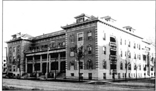
Figure 8. The Colonnade Apartment building as it appeared about 1902. The Lafayette Street balconies of the Altamaha are just visible at the far left of the photo. The streets appear to be unpaved in this view. (Source: Western History / Genealogy Department, Denver Public Library)
