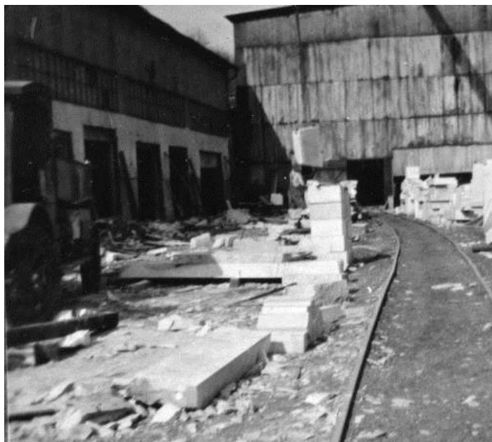
Figure 14. Mead Mill at Marble Quarry, circa 1920s, photographer unknown.
