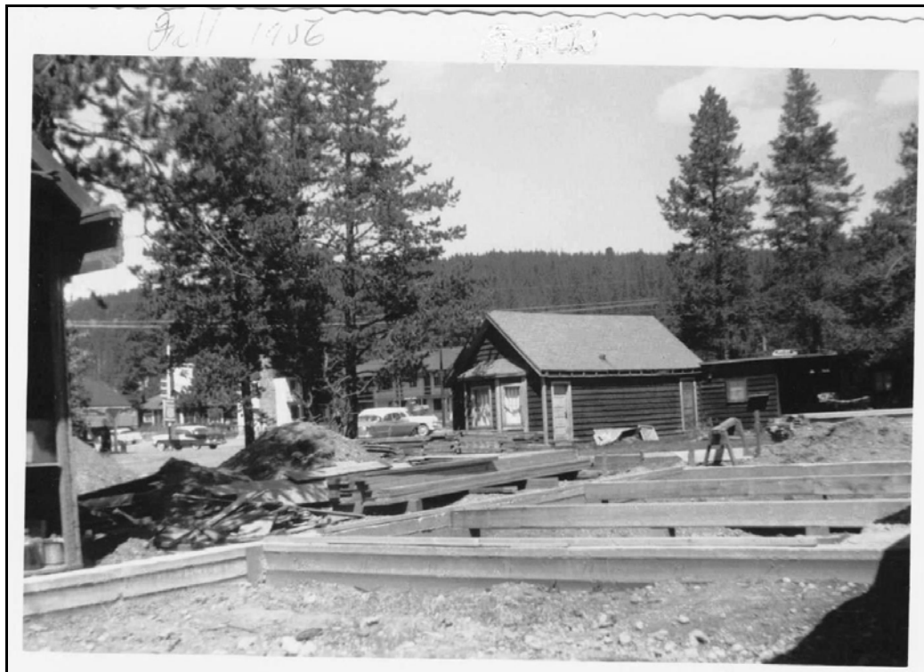
Figure 13. Photo of three-unit cottage court-type building under construction on Smith-Eslick property, Fall 1956
