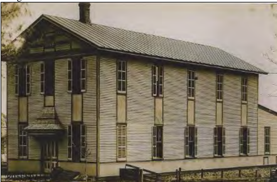
Figure #2: Undated photo (north and west elevations) of the Independent Order of Odd Fellows Lodge No. 89.
