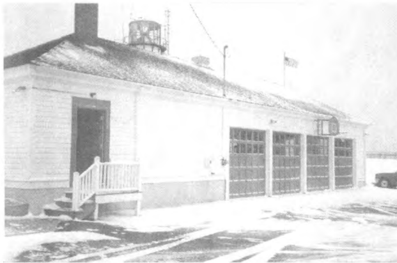
View of garage from 1992, showing new garage doors, ventilating cupola, and infilled opening.
