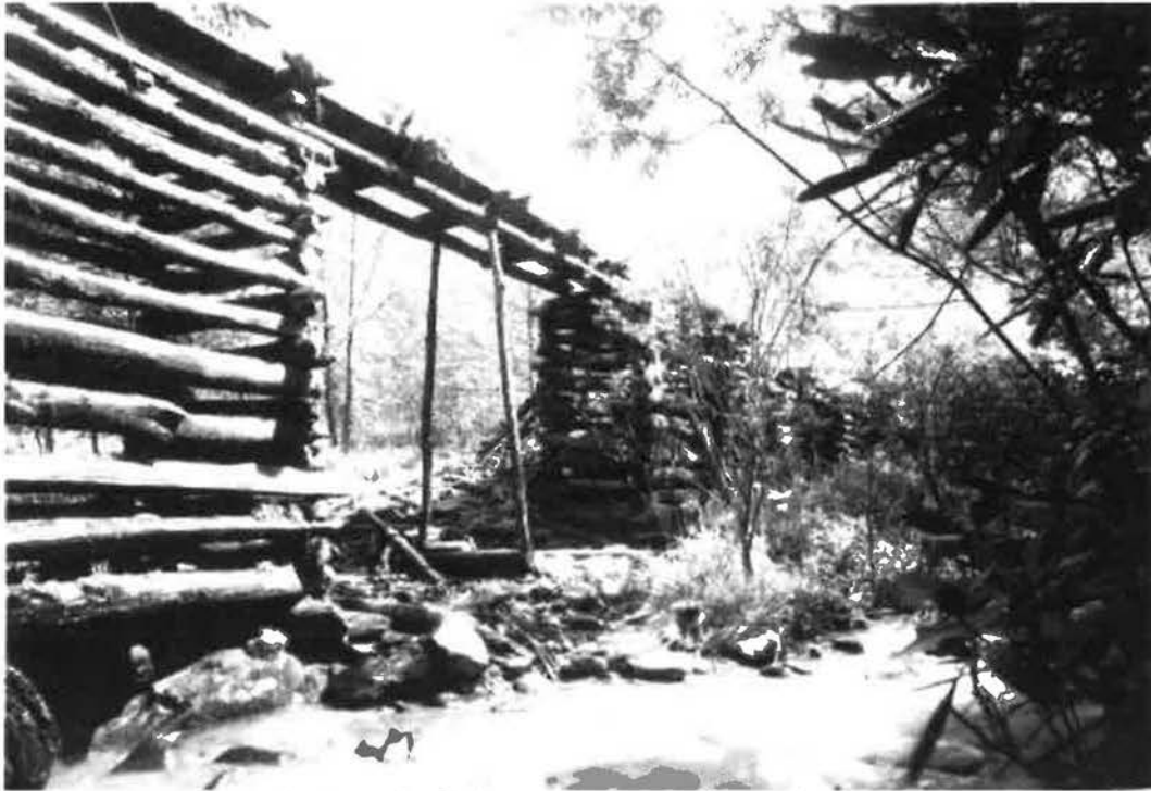
Figure 3. May 1937 photograph of Flume prior to repair, looking west (upstream) toward Mill Race (NPS Neg. No. 3087)
