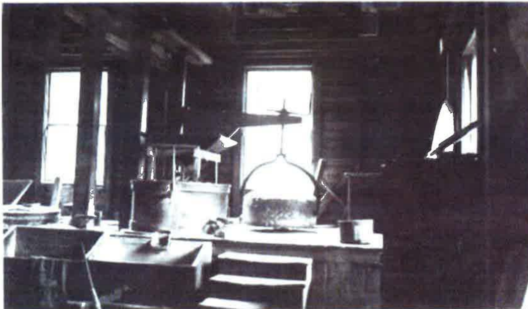
Figure 2. 1935 photograph of first floor of Mingus Mill (NPS Neg. No. 3065).
