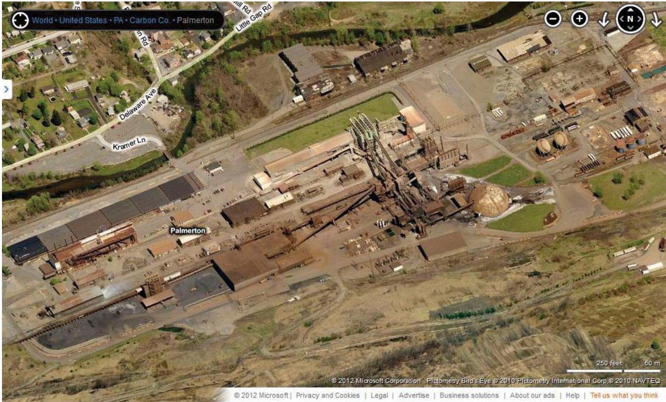
Figure 7 – Aerial view of the East Plant in 2010 (courtesy of Bing Maps).
