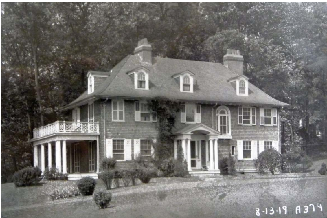
Figure 4 – 355 Columbia Avenue in 1919, after constructon.
