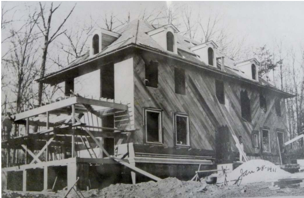
Figure 3 – 355 Columbia Avenue under construction in 1911.
