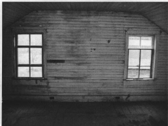
The south bedroom features beaded wallboards; the original 1840s corner stair was removed in the 1890s; the replacement floorboards are visible (right). This room was painted white. Note the "ghost" of the imported Asian floor matting dating from the early 20 th century (R. Jones, 12/2007).
