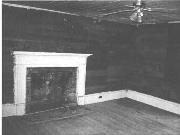
The south parlor retains the 1840s fireplace mantel and evidence of the 1840s corner stair, which was removed during the 1890s renovation and later covered with wallpaper (R. Jones, 12/2007).
