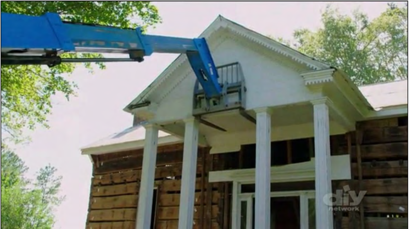
Figure 8: Screenshot of the Removal of the Front Porch of the Noblit-Lytle House, 2017. From “Barnwood Builders” and the DIY Network.
