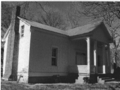
Noblit-Lytle House, looking northwest. (R. Jones, 02/2008).
