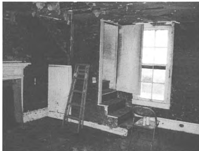
The north parlor retains the 1840s fireplace mantel and 1840s corner stair, including two 1840s 2-panel beveled doors, one leading to the 2 nd floor bedroom and the other to a small closet (R. Jones, 12/2007).
