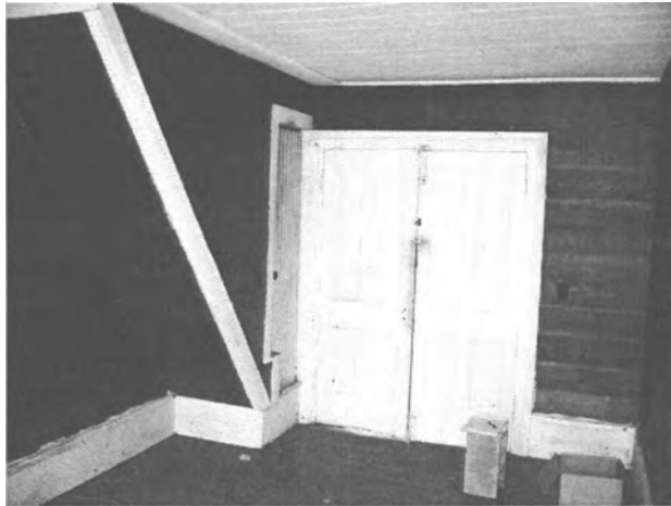
The center hall features a narrow corner stair and double doors (R. Jones, 12/2007).
