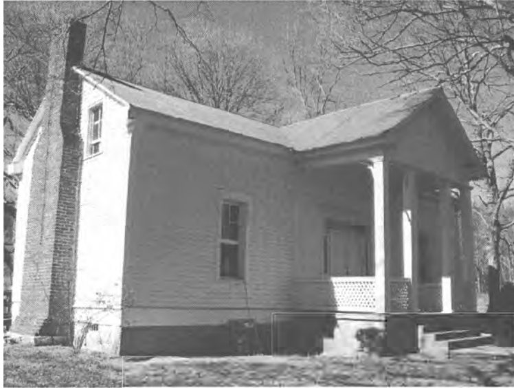
Noblit-Lytle House, looking northwest. (R. Jones, 02/2008).
