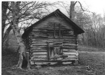
The log smokehouse was constructed in the 19 th century and retains stone chinking (R. Jones, 12/2007).
