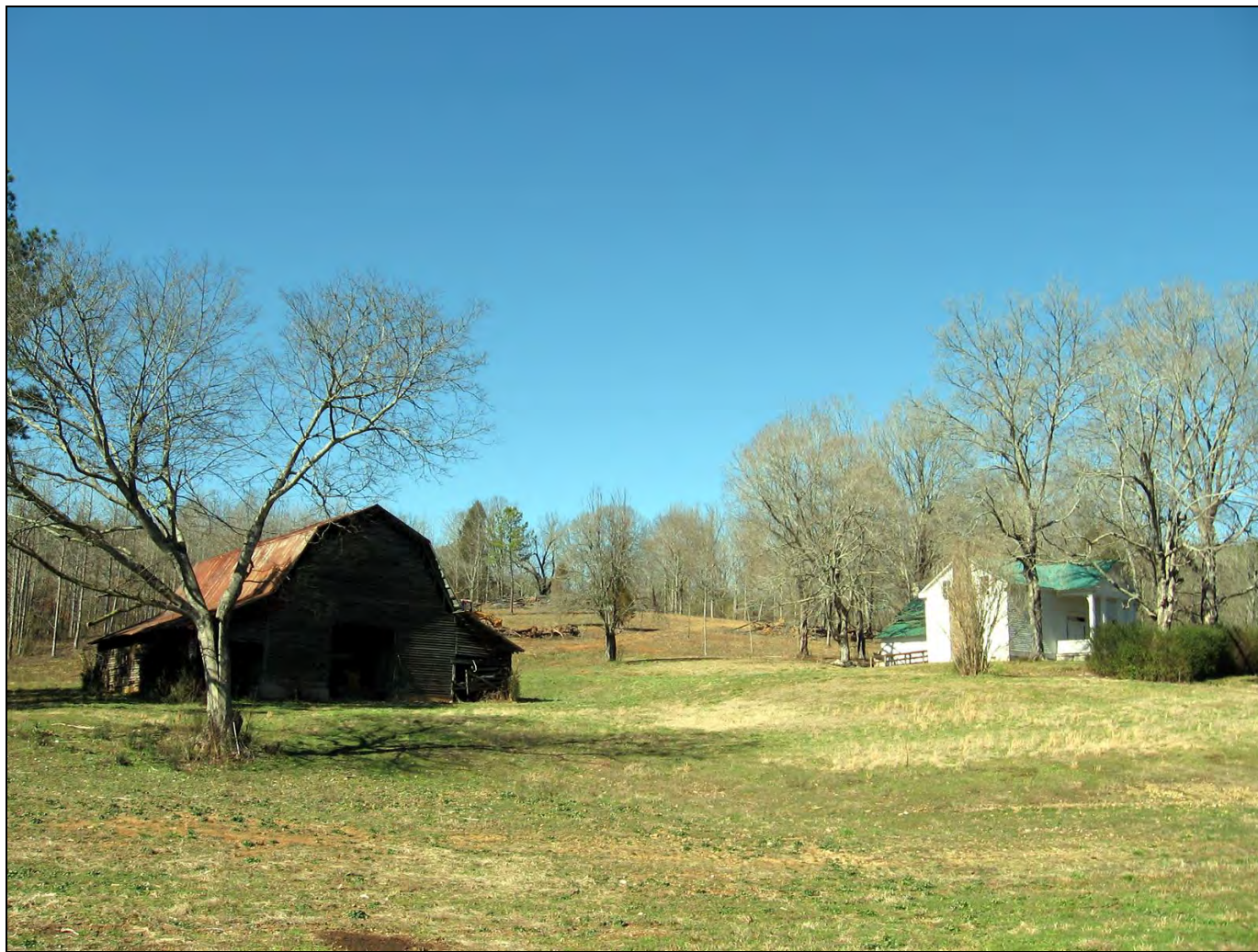
Figure 2: Noblit-Lytle House and Landscape, view to the northwest, from the Noblit-Lytle House National Register Nomination, 2008
