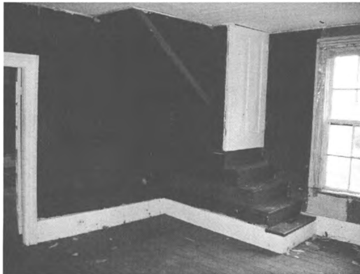
The dining room retains the enclosed corner stair that may have originally been located in the 1890s from the 1840s south parlor; its dimensions match the 1840s north parlor stair (R. Jones, 12/2007).
