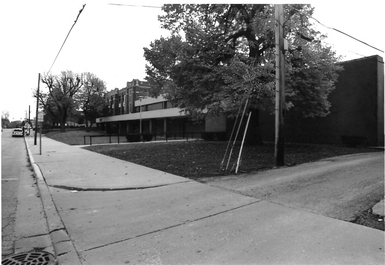
25. Kokomo High School Howard Co., IN FRONT W/ ADDITION
