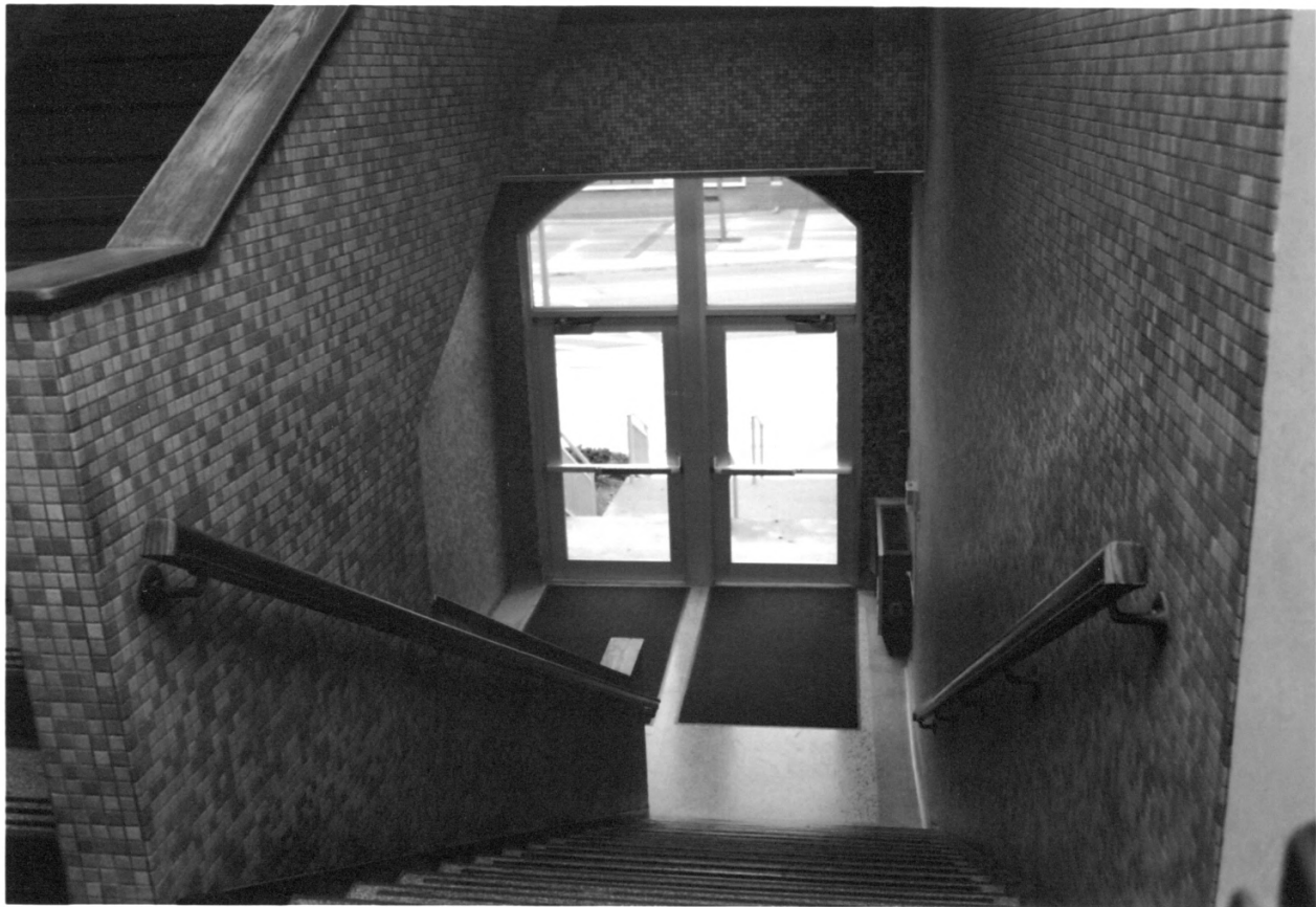
43. Korane High School Howard Co., IN INT. SIDE STAIR, E. ENT.
