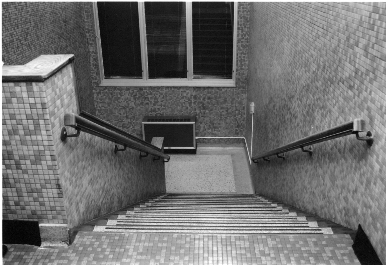
44, KOKOMO HIGH SCHOOL HOWARD Co., IN INT. STAIR E. SIDE
