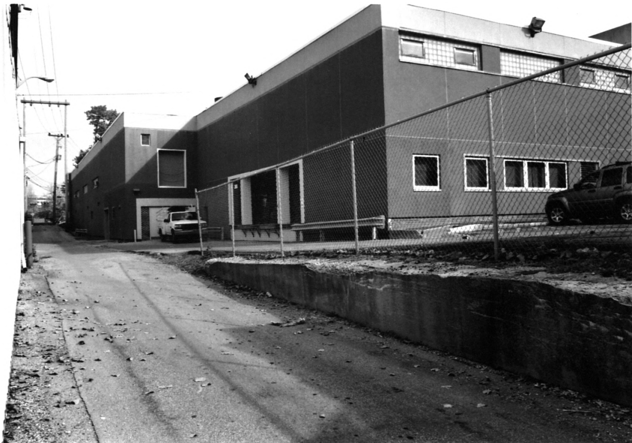
32. Kokomo High School Howard Co., IN Vocational Bldg. Conditions
