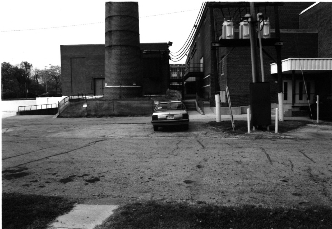
34. Kokomo High School Howard Co., IN BOILER
