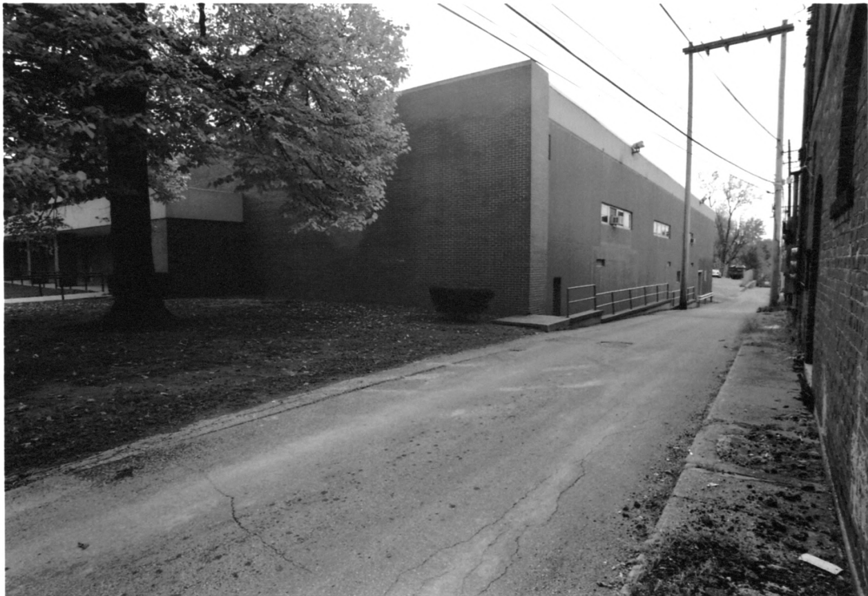
33. KOKOMO HIGH SCHOOL HOWARD CO., IN WEST WALL OF VAC. BLDG.
