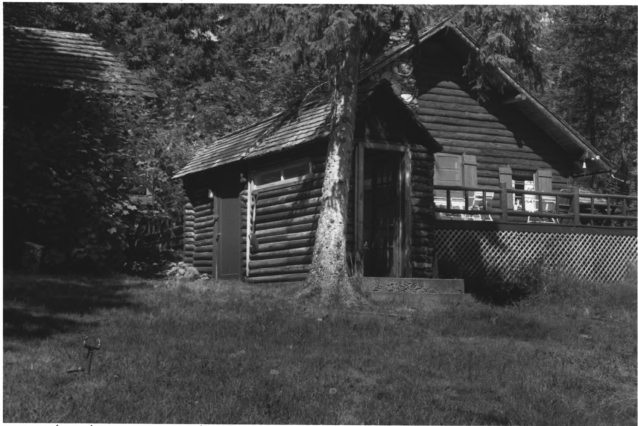
Generator house, Wheeler Camp Glacier National Park, Flathead County, Montana Photograph No. 7
