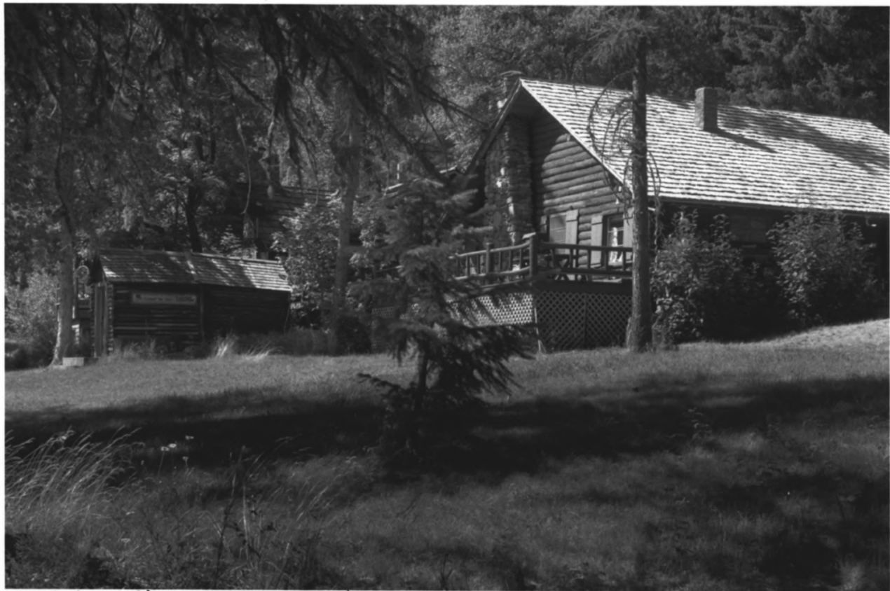
Boys' Cabin (R) and generator house (L), Wheeler Camp Glacier National Park, Flathead County, Montana Photograph No. 6
