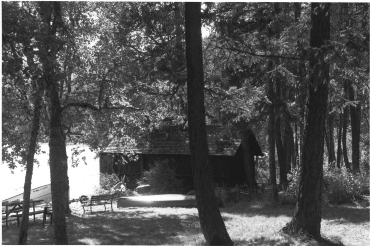
Boathouse, Wheeler Camp Glacier National Park, Flathead County, Montana Photograph No. 2
