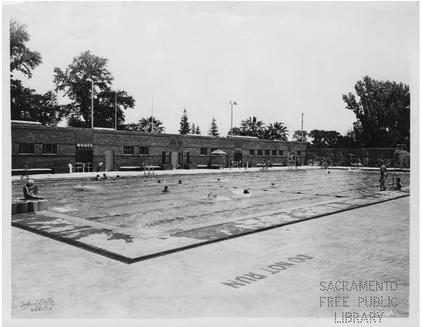
Figure 19. 1937. Pool and bathhouse. Sacramento Public Library.
