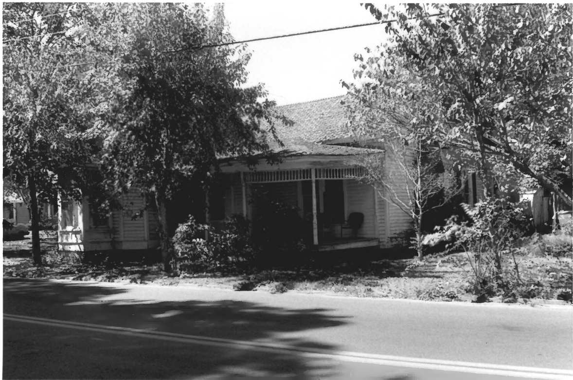
ROSVILLE HISTORIC DISTRICT FAYETTE COUNTY, TN
