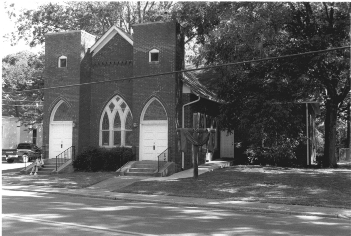
ROSVILLE HISTORIC DISTRICT FAYETTE COUNTY, TN
