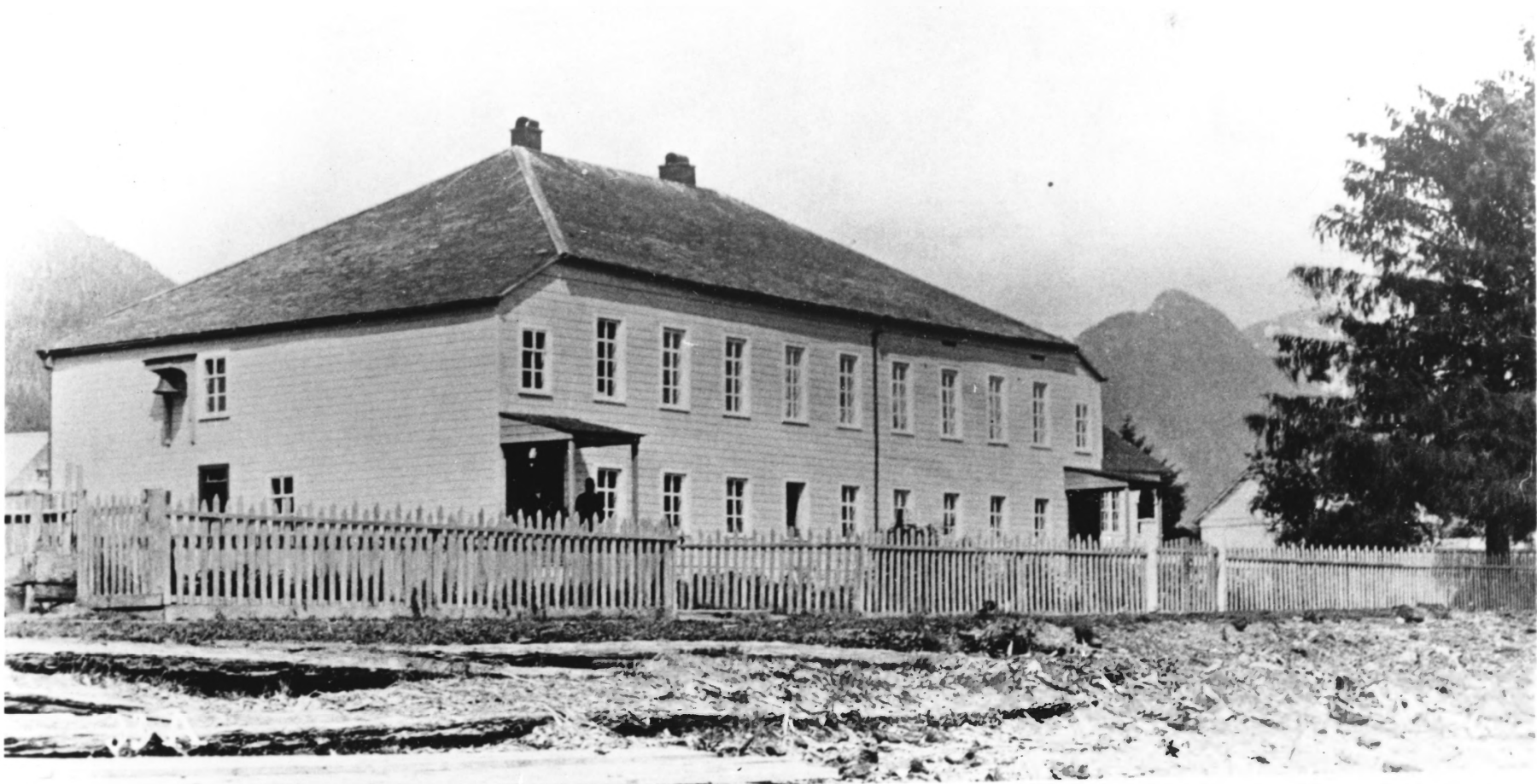
FIGURE #12 . . . SOUTHWEST VIEW OF HOUSE ca. 1890. NOTE RECONSTRUCTED GALLERIES, NEW SIDING AND PORCHES. ALSO NOTE NEW CAP AT EAST CHIMNEY. SITKA NATIONAL HISTORICAL PARK.
