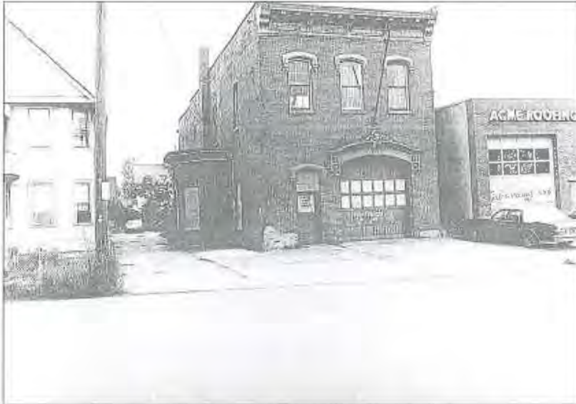
Figure 24.a. Cleveland Fire Engine Company #8, 2599 Scranton, Photo 1988
