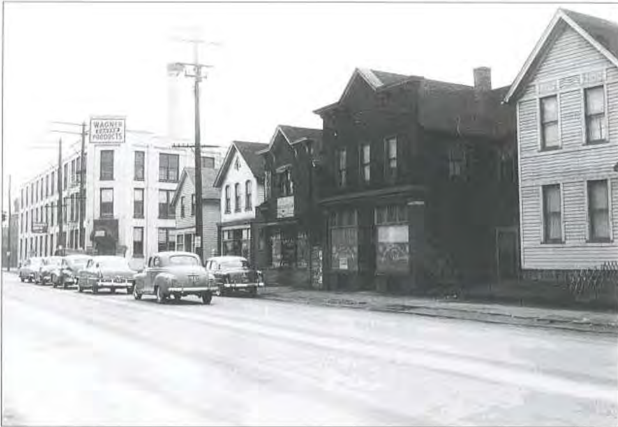
Figure 11. Wagner Awning Building, Starkweather Business District, Photo 1954.
