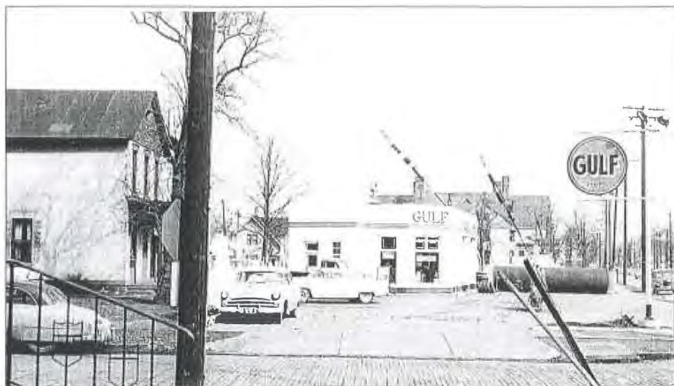
Figure 21.b. F. Dall Gulf Service Station, 2884 Scranton, Photo 1957 Standard box type station used by Gulf in the 1930's. 1
