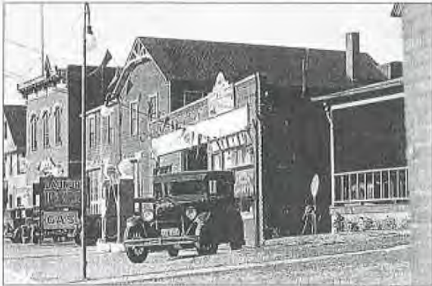
Figure 20.a. Home Family Laundry & Gas Station, 2613-17 Scranton Rd., Photo 1933
