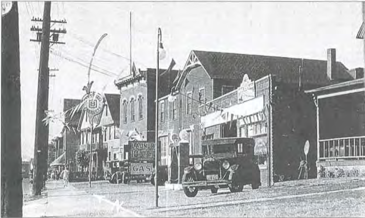
Figure 12. View of Scranton Road, north end, facing northeast including Cleveland Fire Engine Company #8 and Home Family Laundry & Gas Station, Photo 1933
