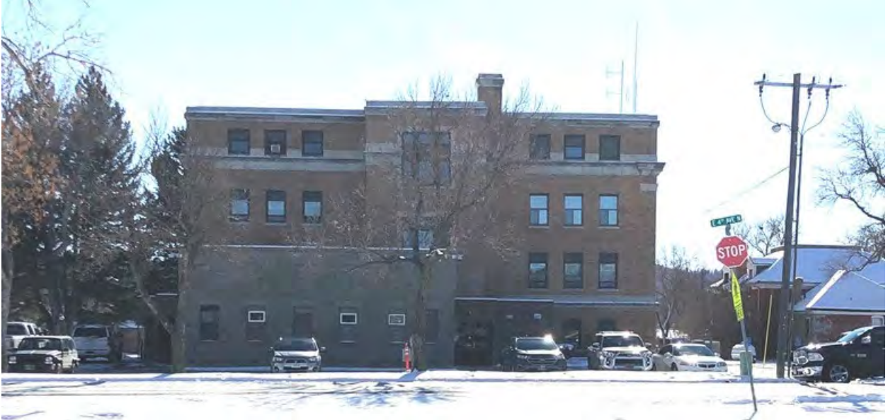
Stillwater County Courthouse, View to the south. North elevation.
