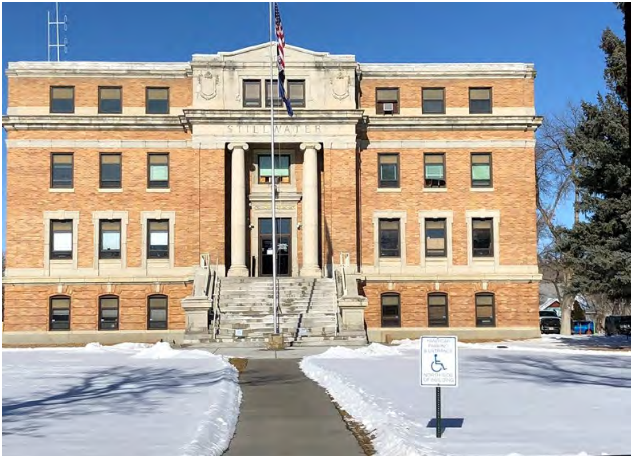
Stillwater County Courthouse, View to the north. South elevation.
