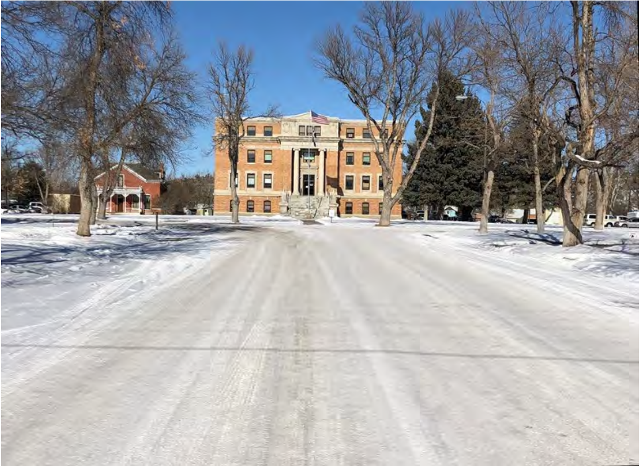
Stillwater County Courthouse, View to the north. South elevation.
