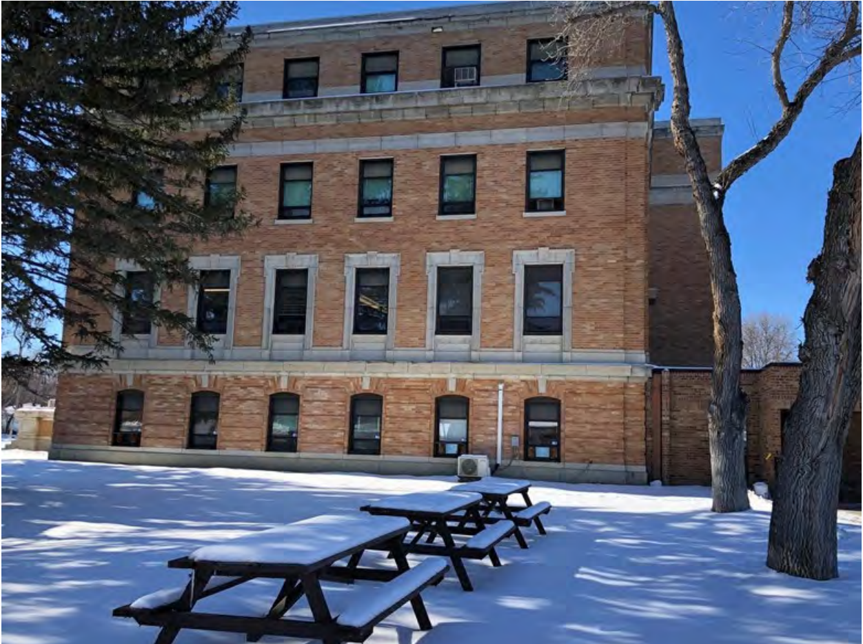
Stillwater County Courthouse, View to the west. East elevation.
