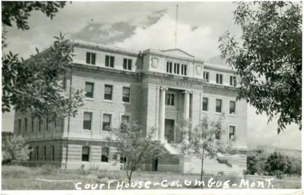
Stillwater County Courthouse, circa 1935. South and west elevations. Courtesy the Museum of the Beartooths, Columbus, Montana.
