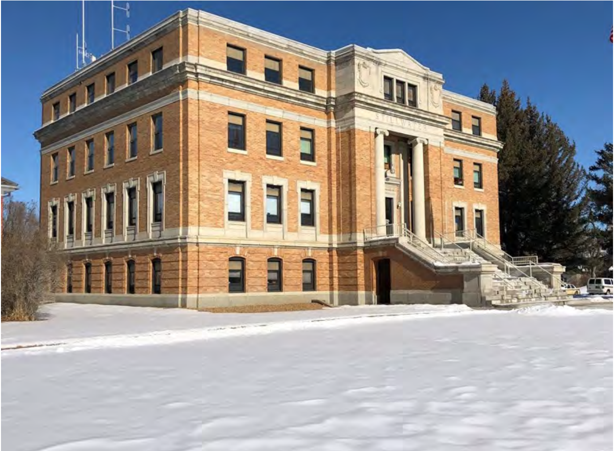
Stillwater County Courthouse, View to the north. South and west elevations.
