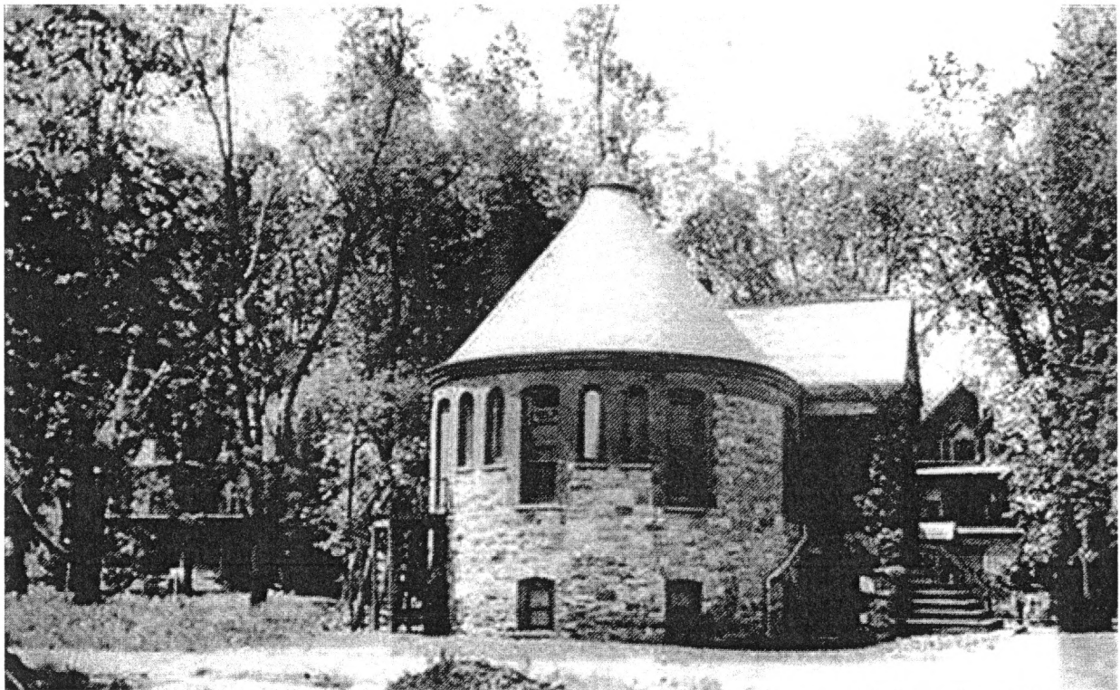
Summit Playhouse, showing east elevation and wood fire escape. Photograph is undated, but likely circa 1918. Note ivy at main elevation. (Courtesy Summit Playhouse Archives.)
