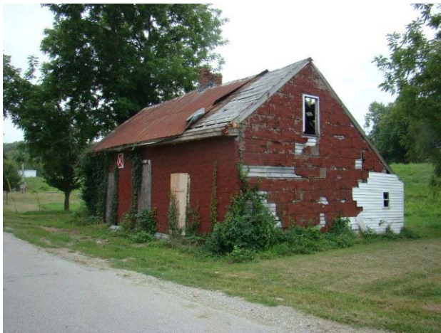
North (front) and west side
