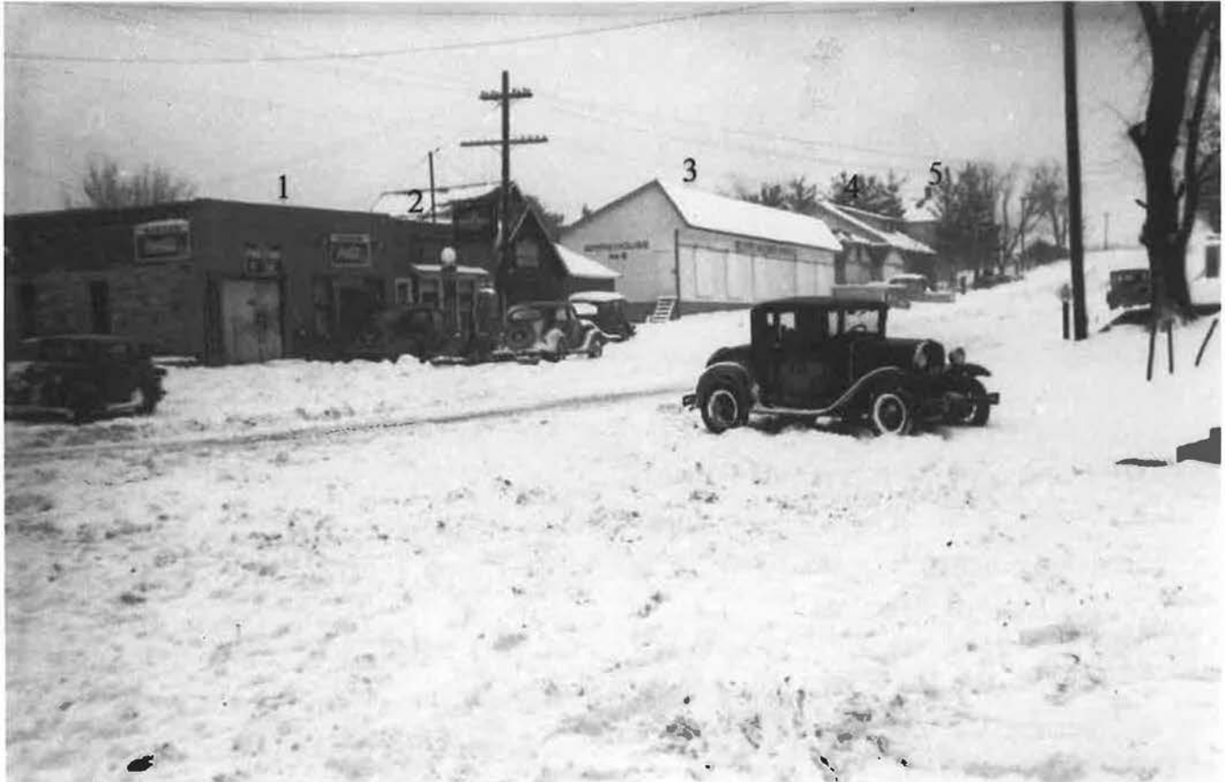
Figure 36. View of Third Street, looking northeast from the southeast corner of Third and Market streets, mid-1930s (before 1936). Left to right: 1) Lange Bros. Shell Service Station and Garage (53-00789); 2) Lange Bros. Store (53-00788); 3) Balster's Warehouse No. 9 (53-00786); 4) Leesekamp House and Garage (53-00785); and 5) the Husmann House (nonextant). The barns between #2 and #3 are nonextant, as is the garage immediately east of Balster's Warehouse No. 9. The other clipped gable garage next to Leesekamp's was a combined dwelling and garage built for Otto Powlishta, who was at the time Scotch Grove's mail carrier. The garage was probably torn down when the gravel drive around the cottages north of these buildings was created. Source: Jean Bohlken Workman, Deltona, Florida
