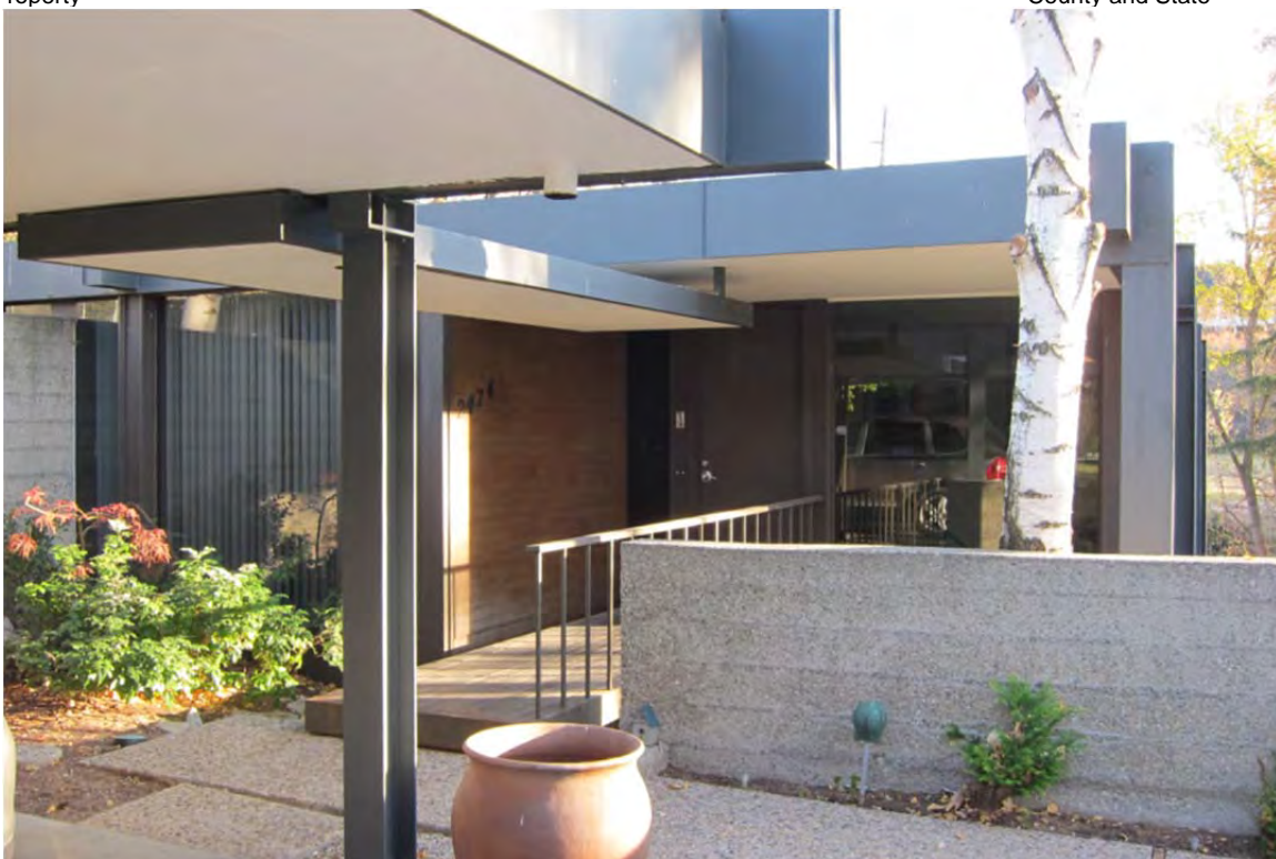
Photograph 7 of 18. View of West Façade stair view detail. Camera facing east.
