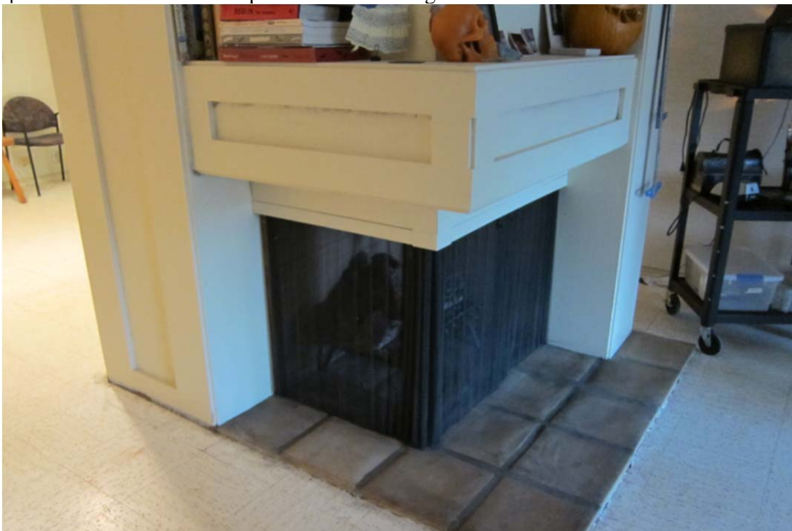
Photograph 14 of 18. Downstairs fireplace. Camera facing northeast.
