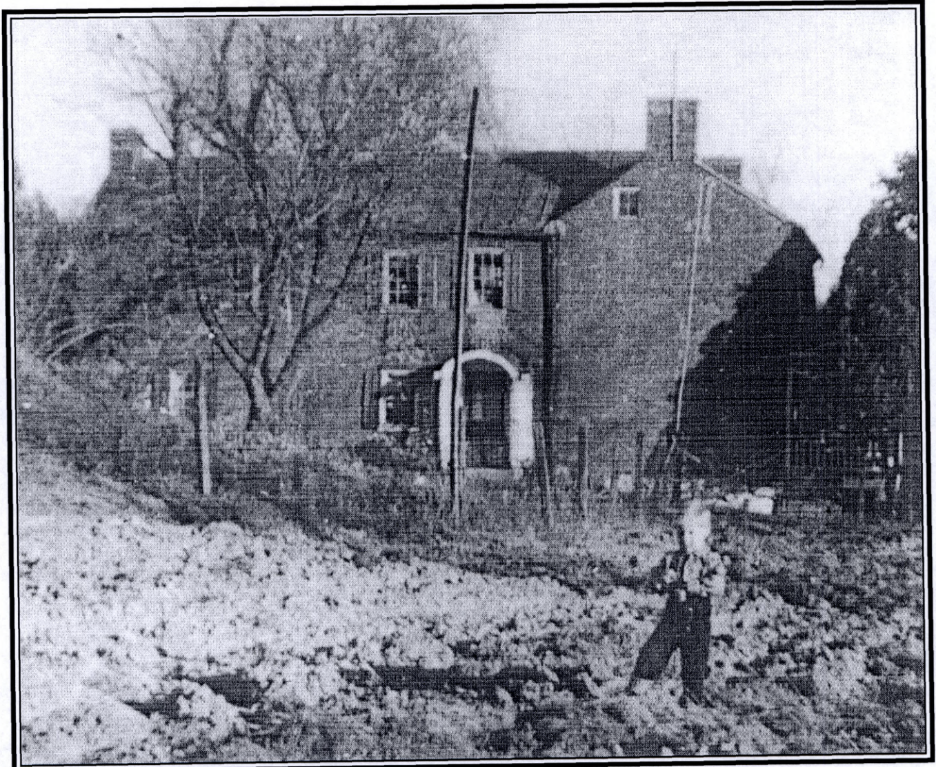
Fig. 2 By the time of this photo, the porticos seen in Fig. 1 had been replaced. The portico on the facade was replaced by a substantial porch, while that on the west elevation was replaced by a semi-circular hood.
