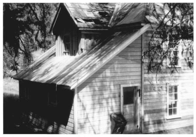
District. Vicinity Granite, Oregon 3. Photographer: Unknown 4. Date of Photograph: 8/78 5. Location of Negative: Dale Ranger Station, Dale, Oregon 97880 Looking northeast, rear elevation of Residence # 1092, showing deteriorated roof materials on added central dormer.
