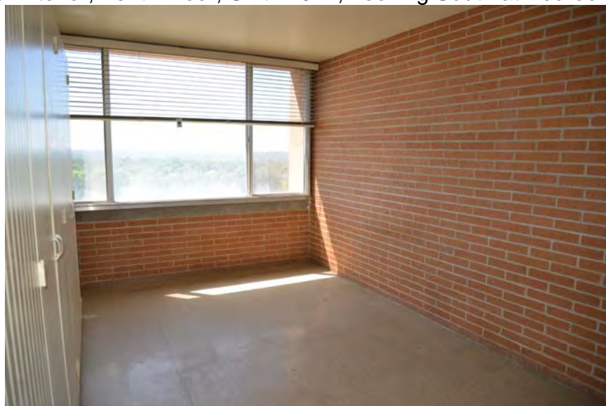
Photo 18. Interior, Tenth Floor, Unit #1017, Looking South at Bedroom, Typical
