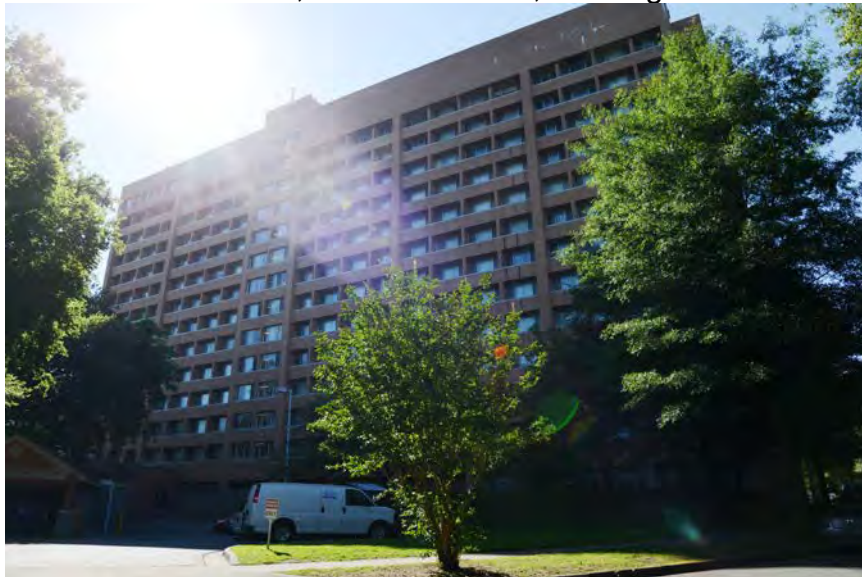
Photo 4. Exterior, North Elevation, Looking Southeast
