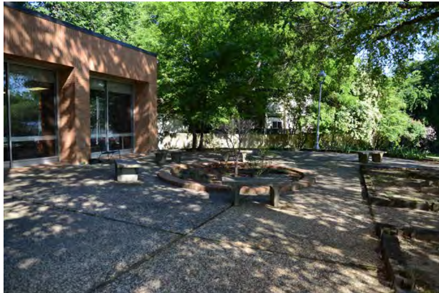
Photo 6. Site and East Elevation of Community Room, Looking Northwest
