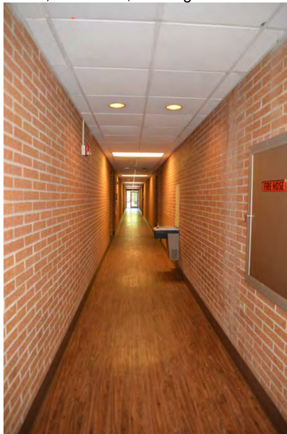
Photo 12. Interior, First Floor, Looking West at Corridor, Typical
