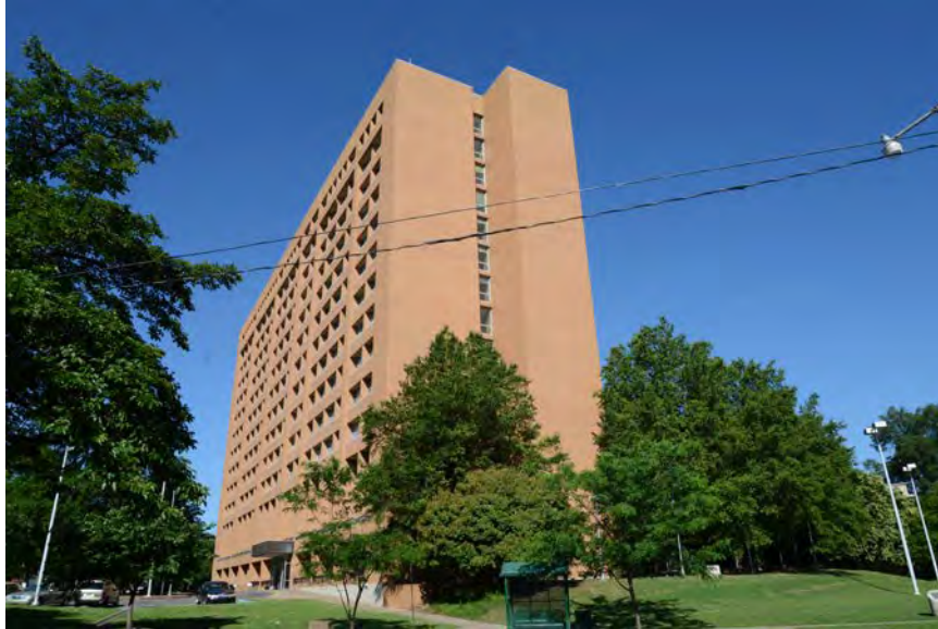
Photo 3. Exterior, South and East Elevations, Looking West
