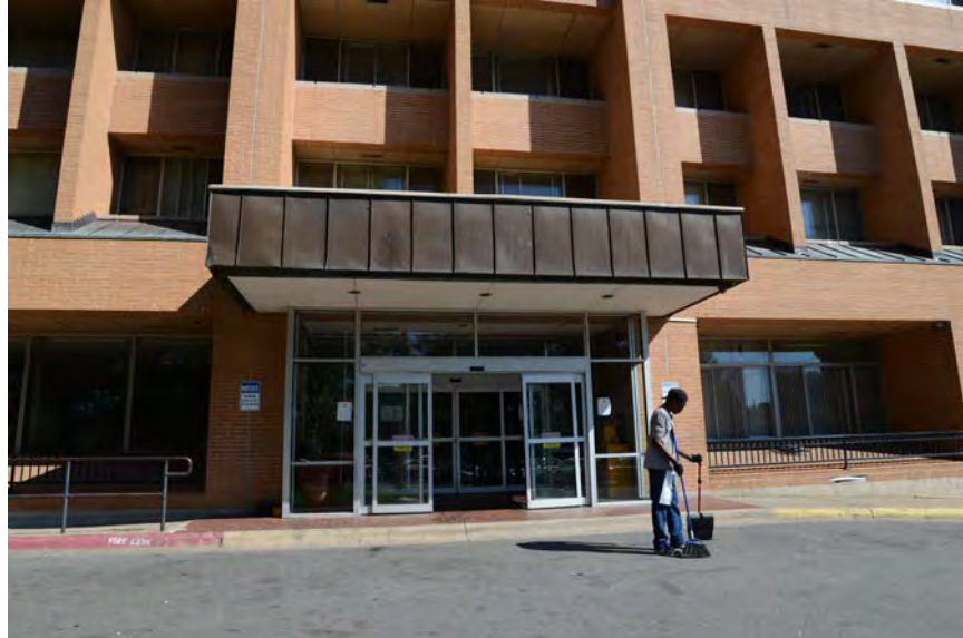
Photo 9. Exterior, South Elevation, Looking Northwest at Entrance
