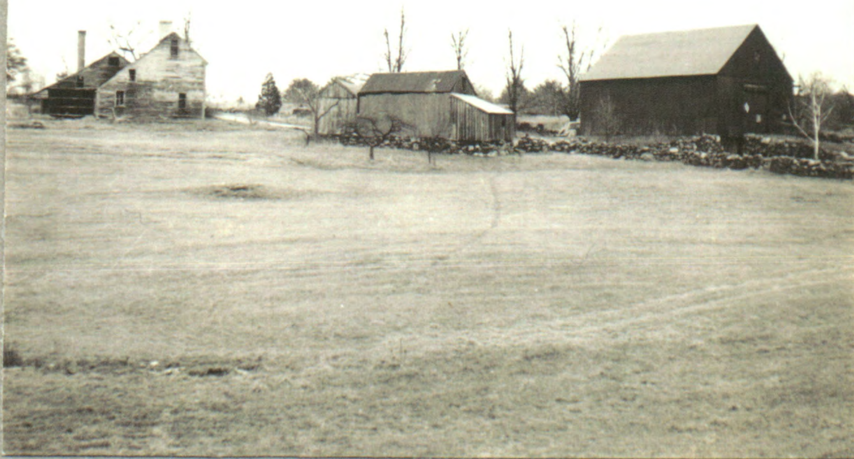
Three Building w View
