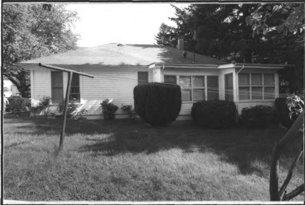
Building 51 is a one story, wood frame building with a hip roof. The building measures 47 feet by 47 feet. The siding is 6 inch drop siding with trim boards. Windows are wood sash and frame double-hung windows with 6 over 2 lights.
