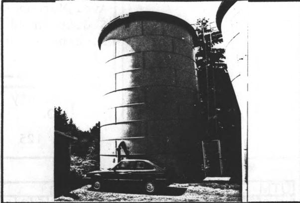
Structure 125 is a cylindrical steel fresh water tank measuring 30 feet in diameter and 40 feet in height. The construction is of riveted steel plate with a conical shingled roof. Originally constructed in 1896 to provide fresh water to the Naval Shipyard. The tank was relocated in 1918 for the construction of Structure 314, a larger fresh water tank.
