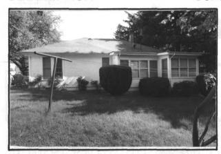
Building 51 is a one story, wood frame building with a hip roof. The building measures 47 feet by 47 feet. The siding is 6 inch drop siding with trim boards. Windows are wood sash and frame doublehung windows with 6 over 2 lights.
