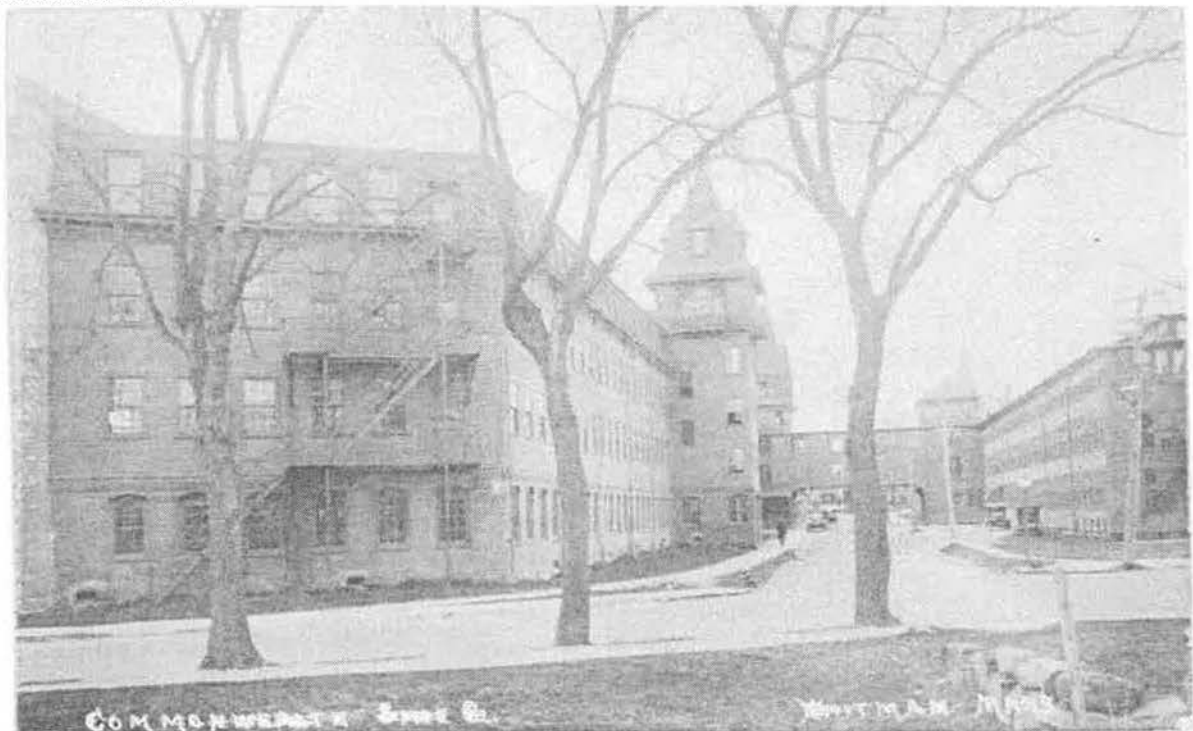
Figure 2b. Undated. View north. Building 1 at left, Building 2 at right. Two-story connector at center. After 1919.
