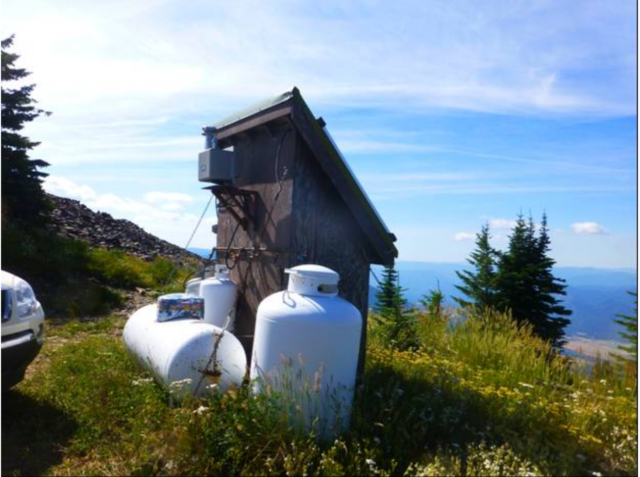
MT_SandersCounty_CougarPeakLookout_0005. Looking west to the radio repeater shed.
