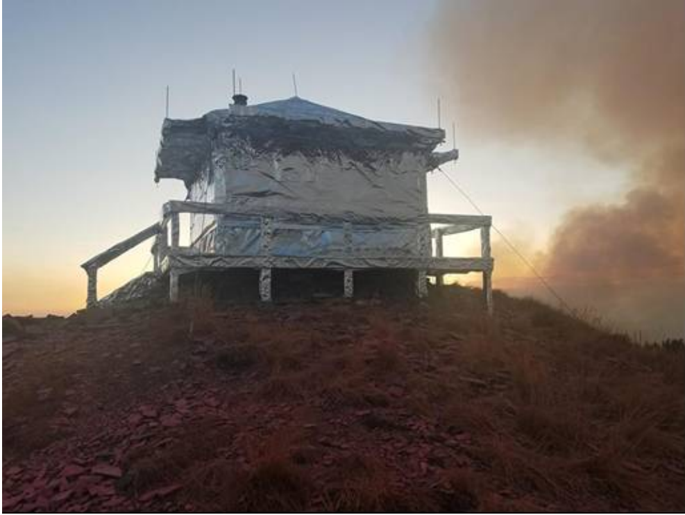
Figure 2. Cougar Peak Lookout wrapped in "cabin wrap."
