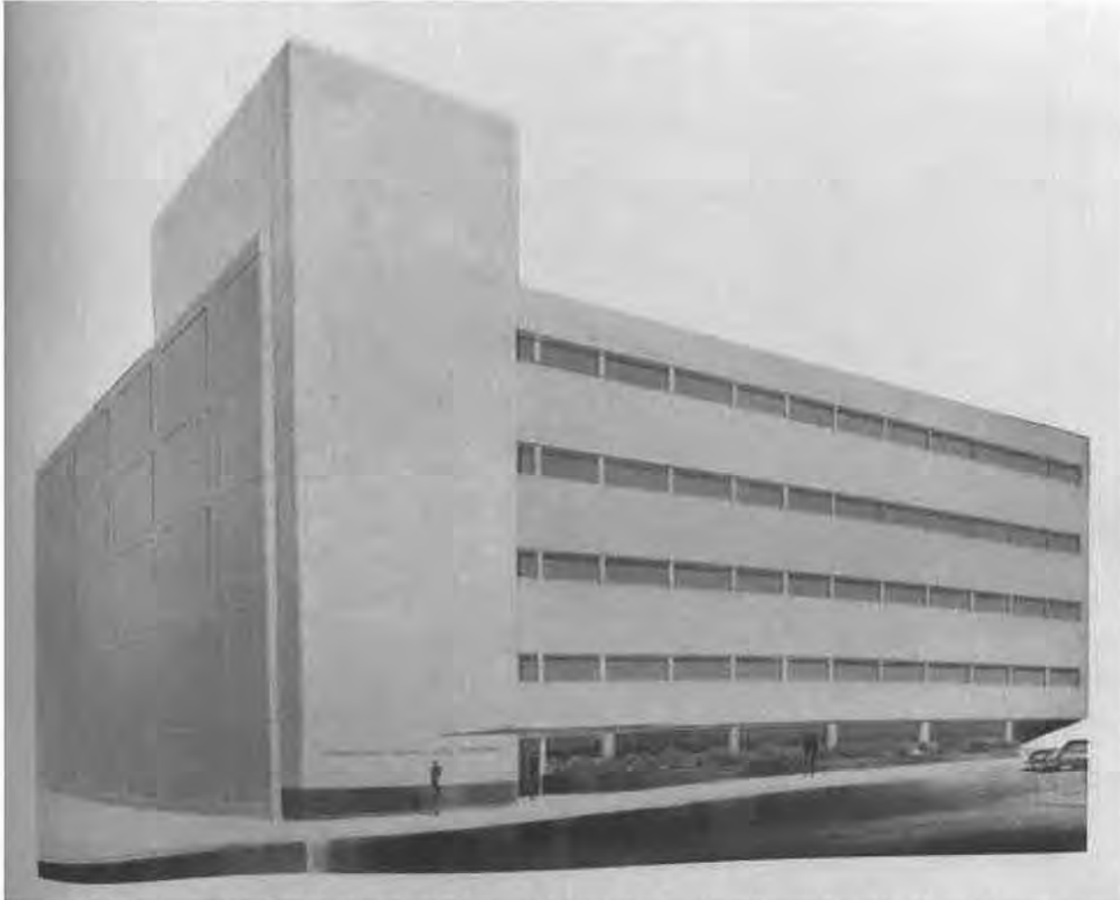
Figure 12. Image of original design for Minnesota Mutual's new building. "New Building Plans Announced," Application (Official Publication of the Minnesota Mutual Life Insurance Company Saint Paul, Minnesota) , September 1950, Minnesota Historical Society Collections.
