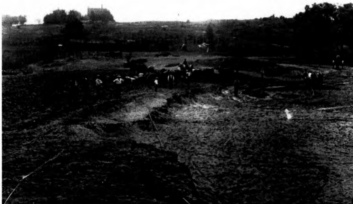
Seaside Park under construction c. 1905. Collection of the Marblehead Department of Recreation and Parks.
