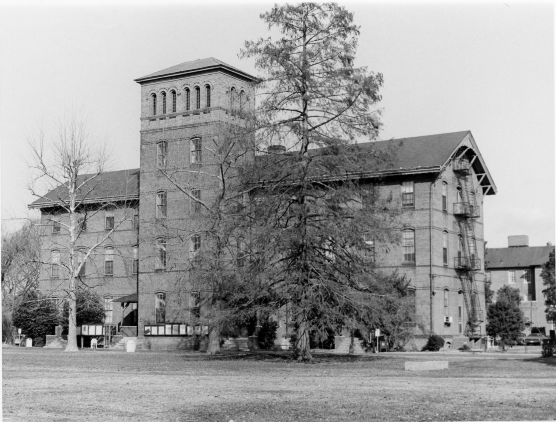
Stone Building, Hampton Institute, Hampton, Virginia
