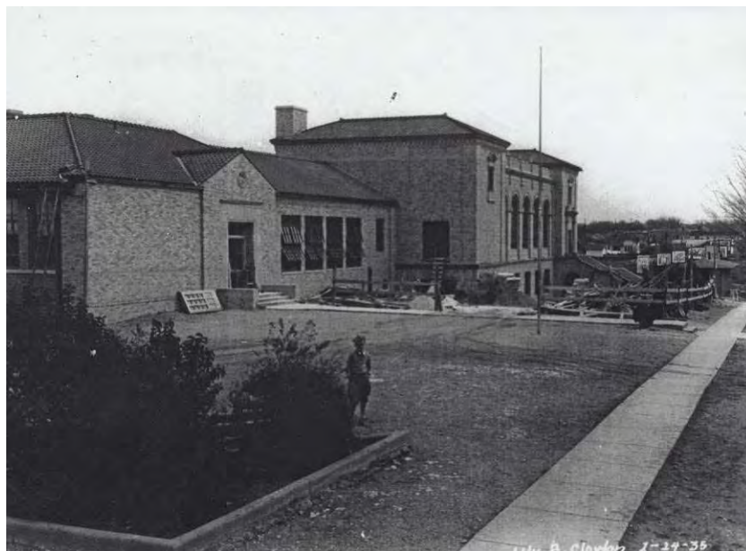
Figure 4: Looking northeast at renovated façade of the 1922 school and the 1934-1935 addition. Photo dated January 24, 1935. Courtesy Lily B. Clayton Archives.
