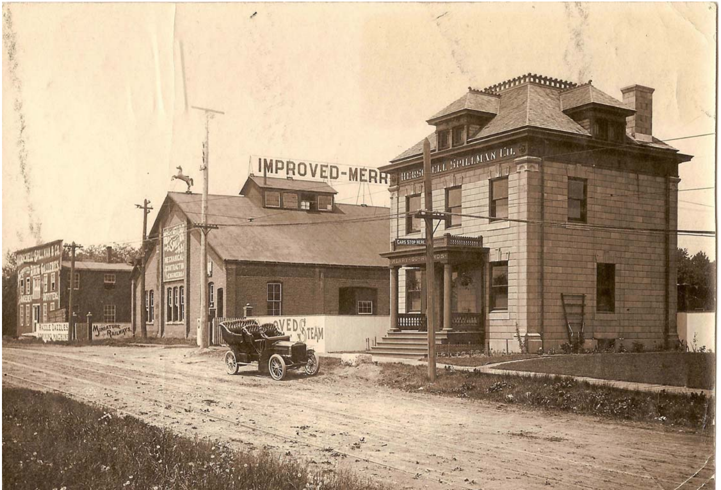
Photo looking northwest along Sweeney Street showing the Herschell-Spillman Company buildings. Note administration building (demolished) in the foreground, and ca. 1895 Power House building in the middle. Photo taken ca. 1910.
