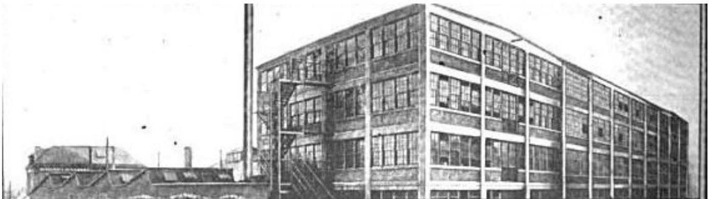
Looking southwest showing ca. 1913 and ca. 1917 concrete frame additions. Note buildings in foreground. Photo published in Automotive Industries , March 7, 1918.
