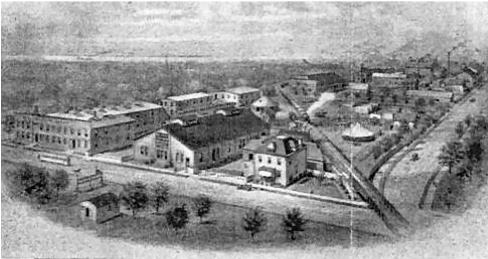
Historic Photo taken ca. 1900 of ca. 1895 Herschell-Spillman Motor Company Complex looking northwest.
