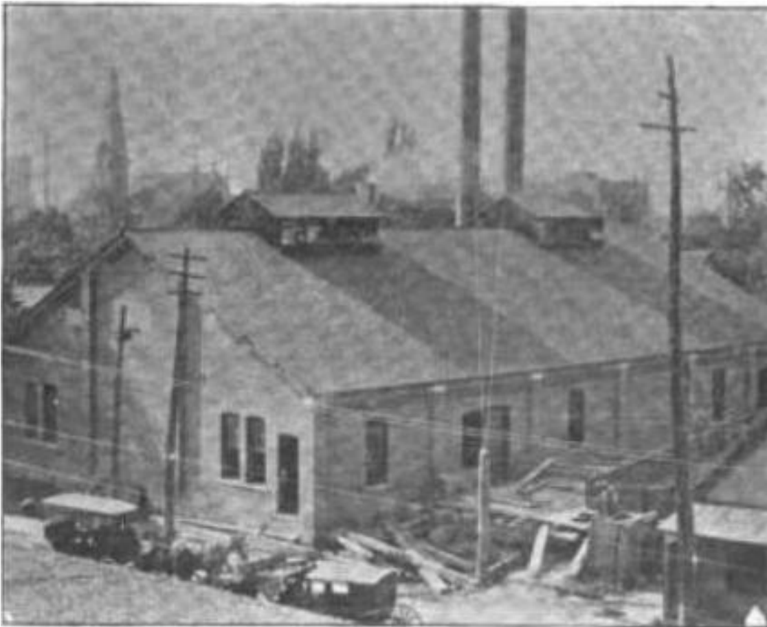
Historic Photo of ca. 1895 Power House looking northwest. Photo published in Electrical Engineer , 1895.
