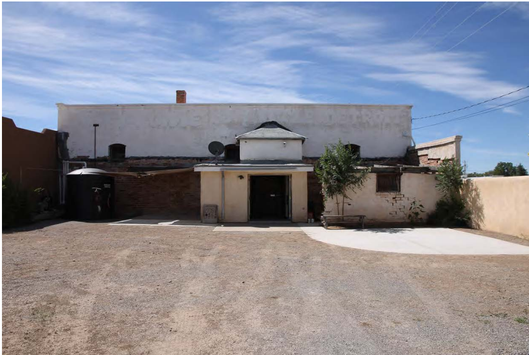
Rear elevation with elevator tower, photographer facing south.
