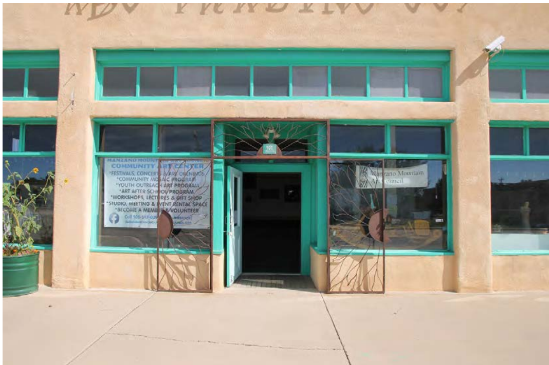
2. Detail of main entrance, photogrpaher facing north.
