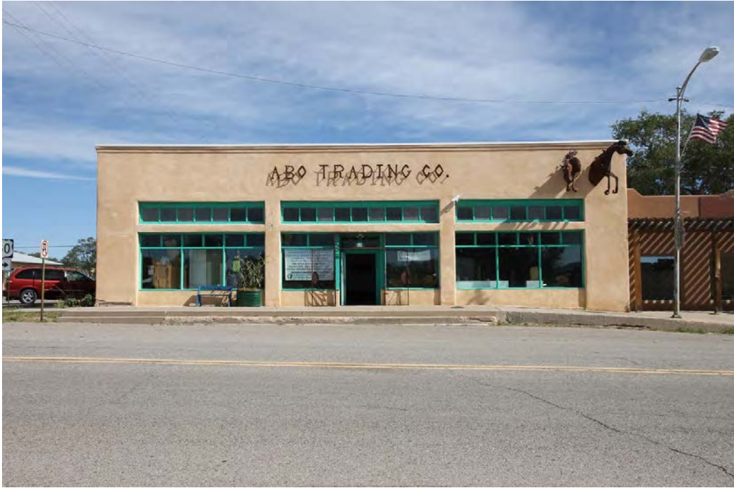
1. Main (south) façade, photogrpaher facing north.
