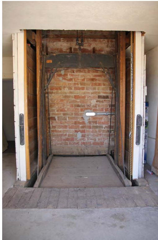
13. Interior, freight elevator, photographer facing south.
