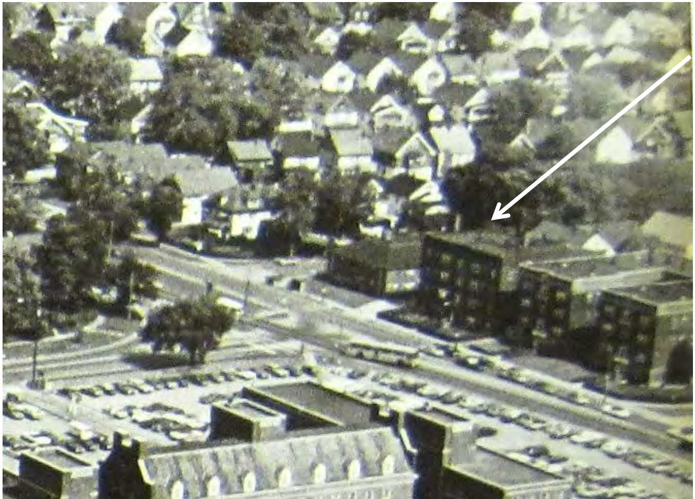
Figure 14: East Boulevard Apartment House, 1975 Indicated by arrow
