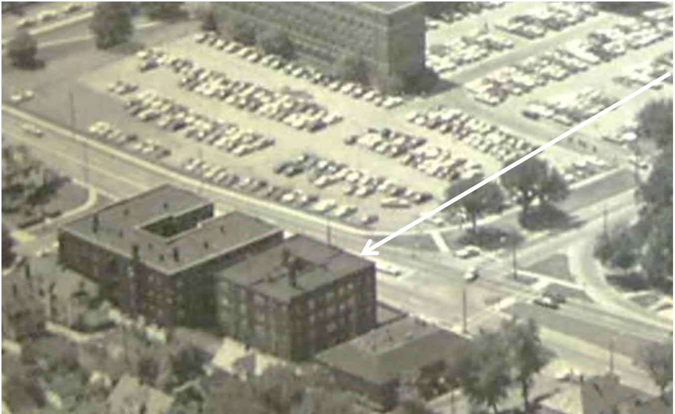
Figure 13: East Boulevard Apartment House, 1975 Indicated by arrow
