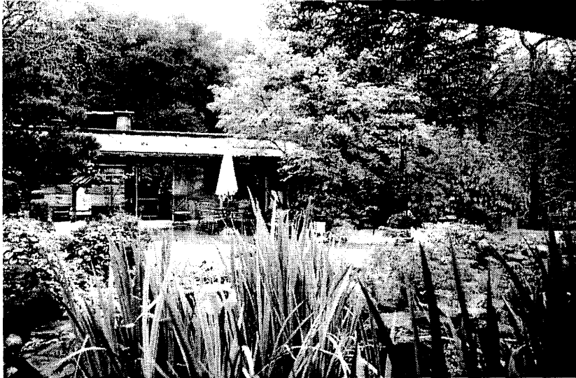
Figure 7. The Guest House, view southwest, looking across the Koi pond (swimming pool) from the bedroom wing of the house.
