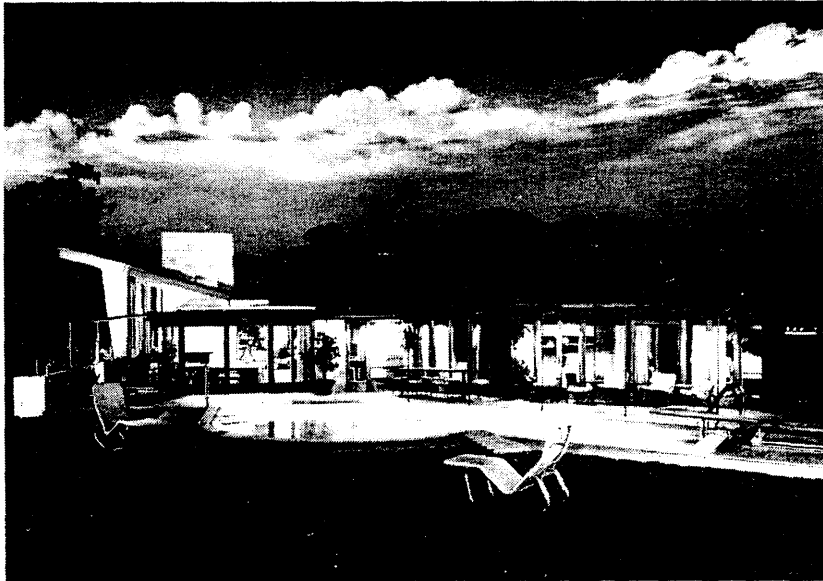
Figure 1. Rear Elevation circa 1951, view north. Photographer: Maynard Buehler.
