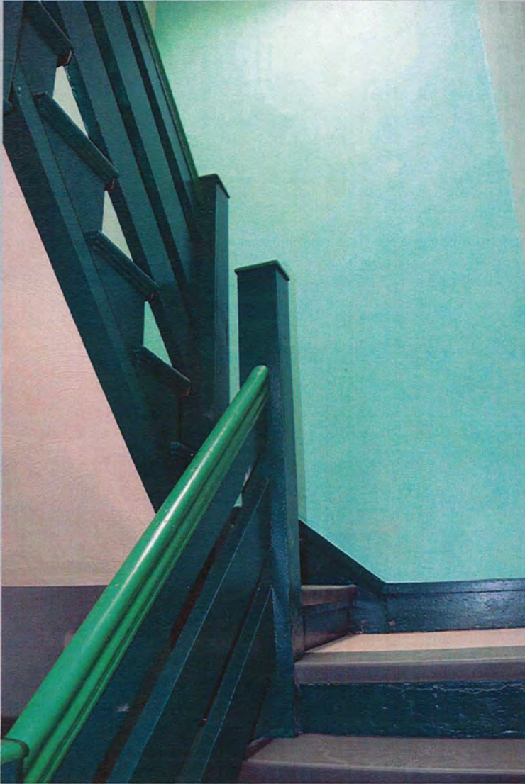
9. 103 Norfolk Street, second floor stair, looking southeast
