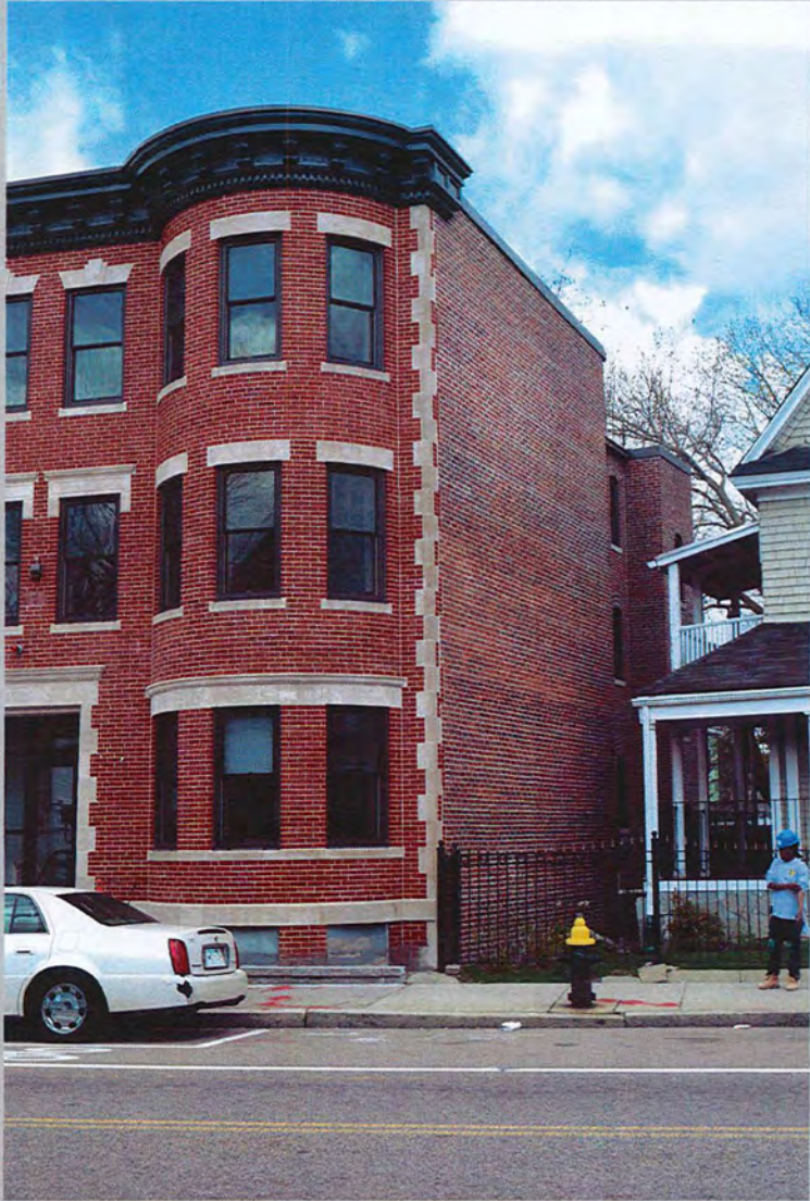
5. 97 Norfolk Street, east elevation looking northwest
