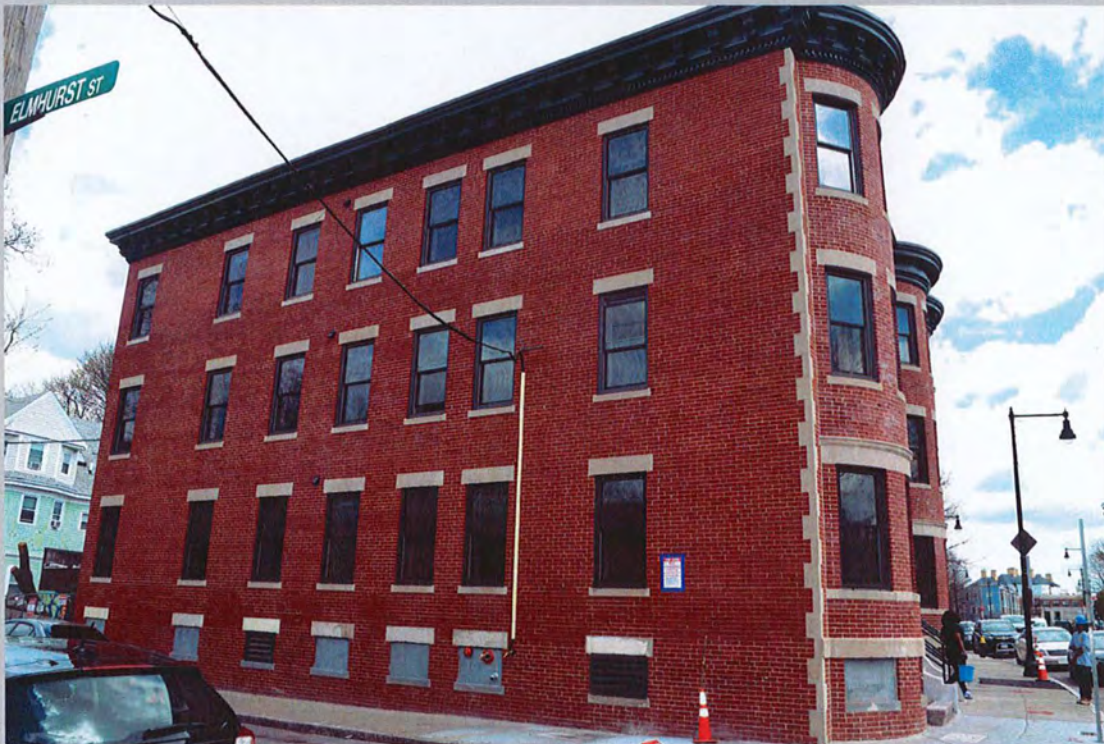
4. Elmhurst Street (west) elevation, looking northeast
