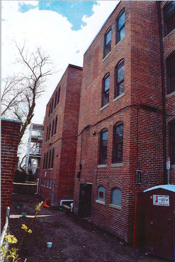
7. Detail north elevation, looking southeast
