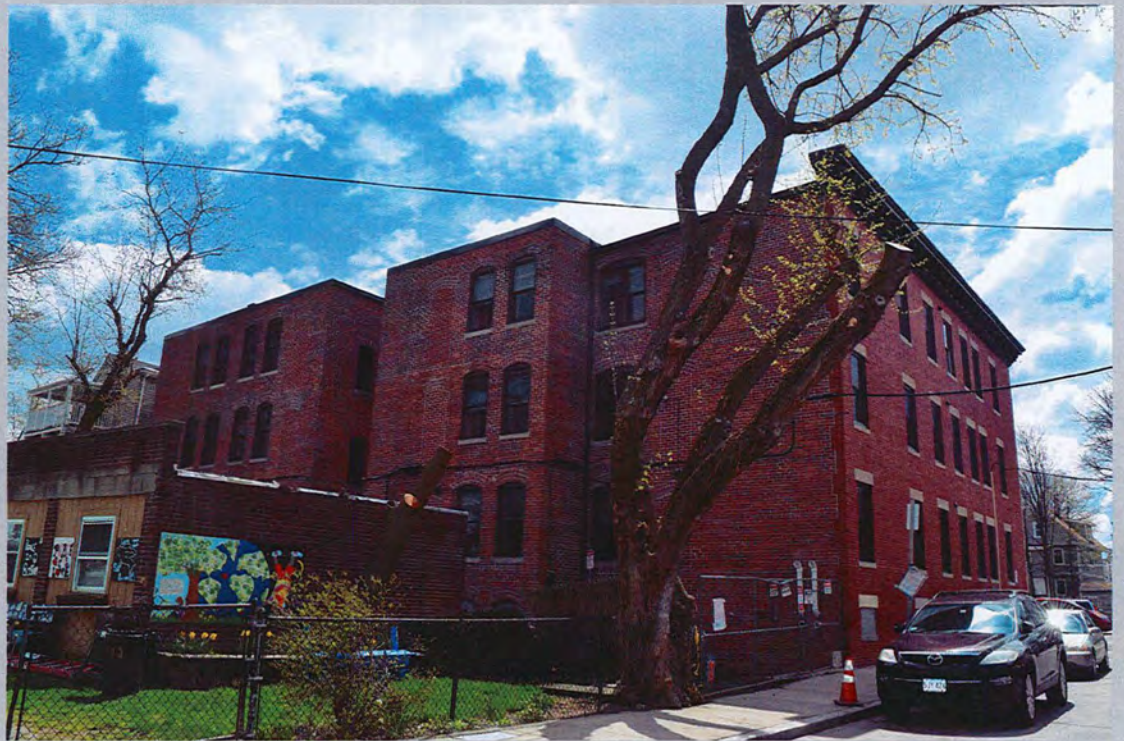
6. 97-103 Norfolk Street, north elevation, looking southeast
