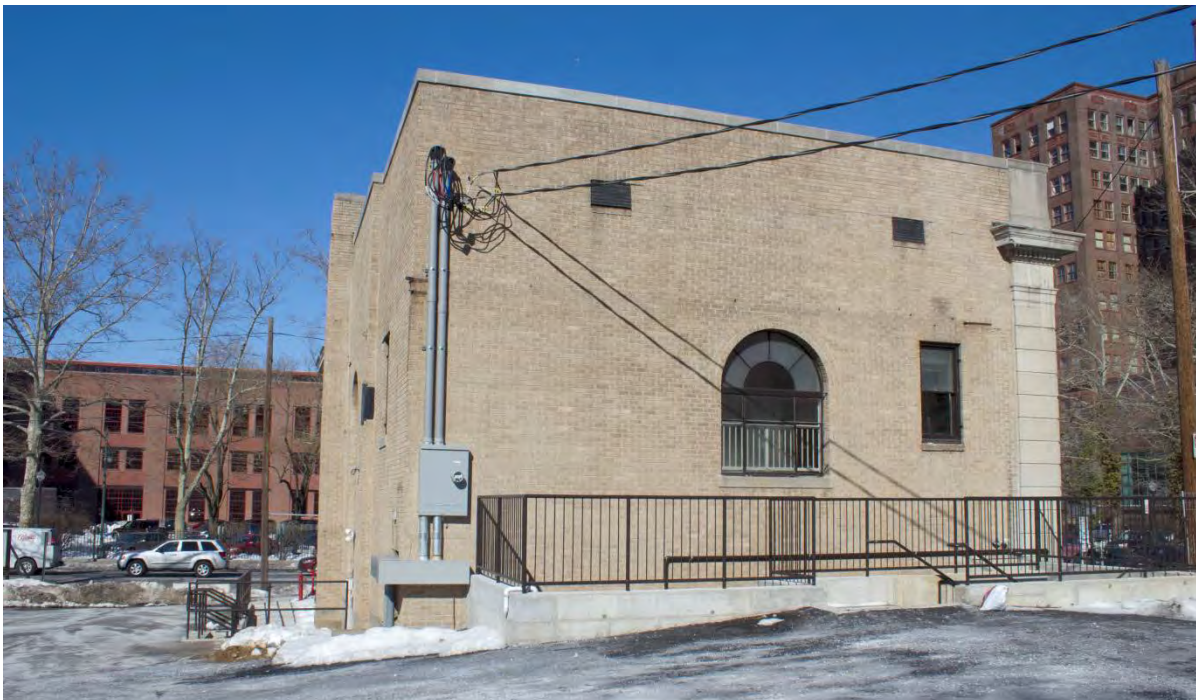
Photo 4—Rear elevation, camera facing N; new delivery entrances to kitchen and basement hidden by low concrete block wall and railing.
