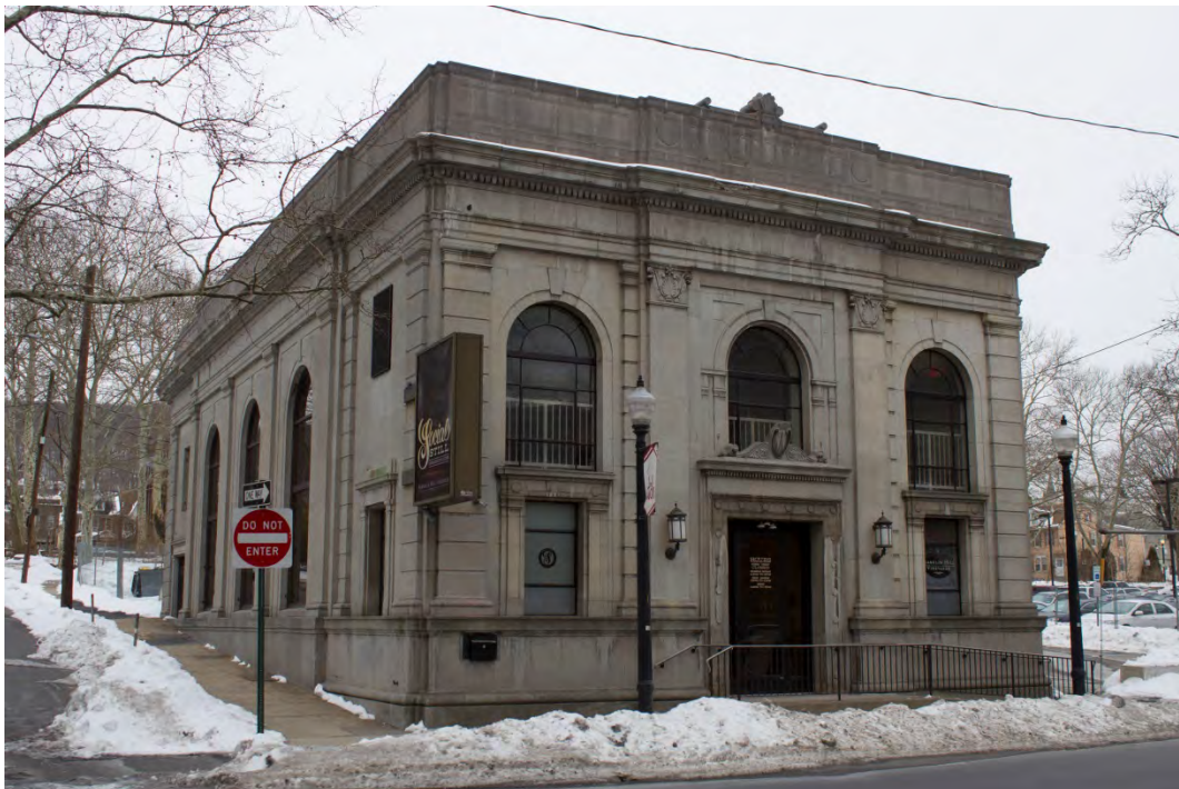
Photo 2—Street-side facades from corner of 3 rd and Pierce Streets, facing SW
