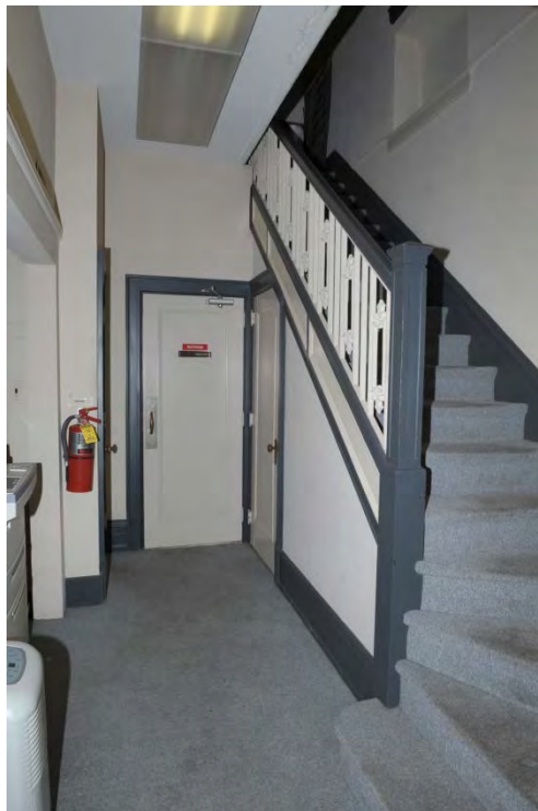
Photo 14—Interior, stairway to south mezzanine (pre-rehab); facing SW.
