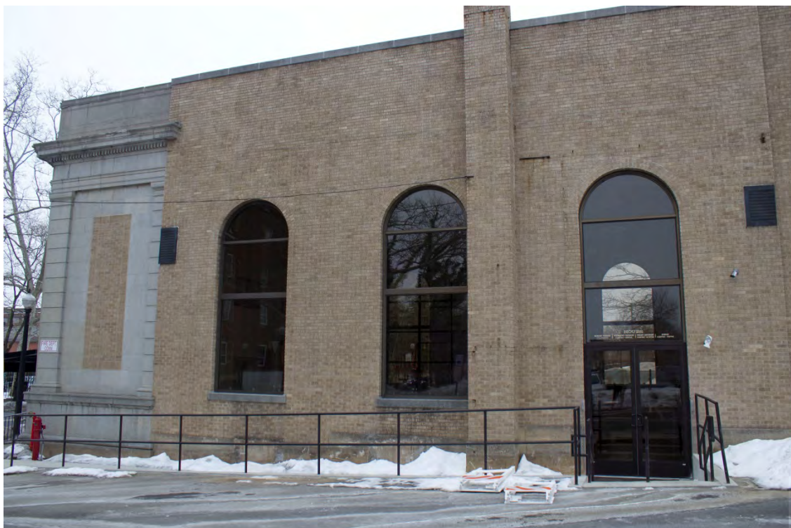
Photo 6—West elevation, facing E, showing converted window bay to create doorway.
