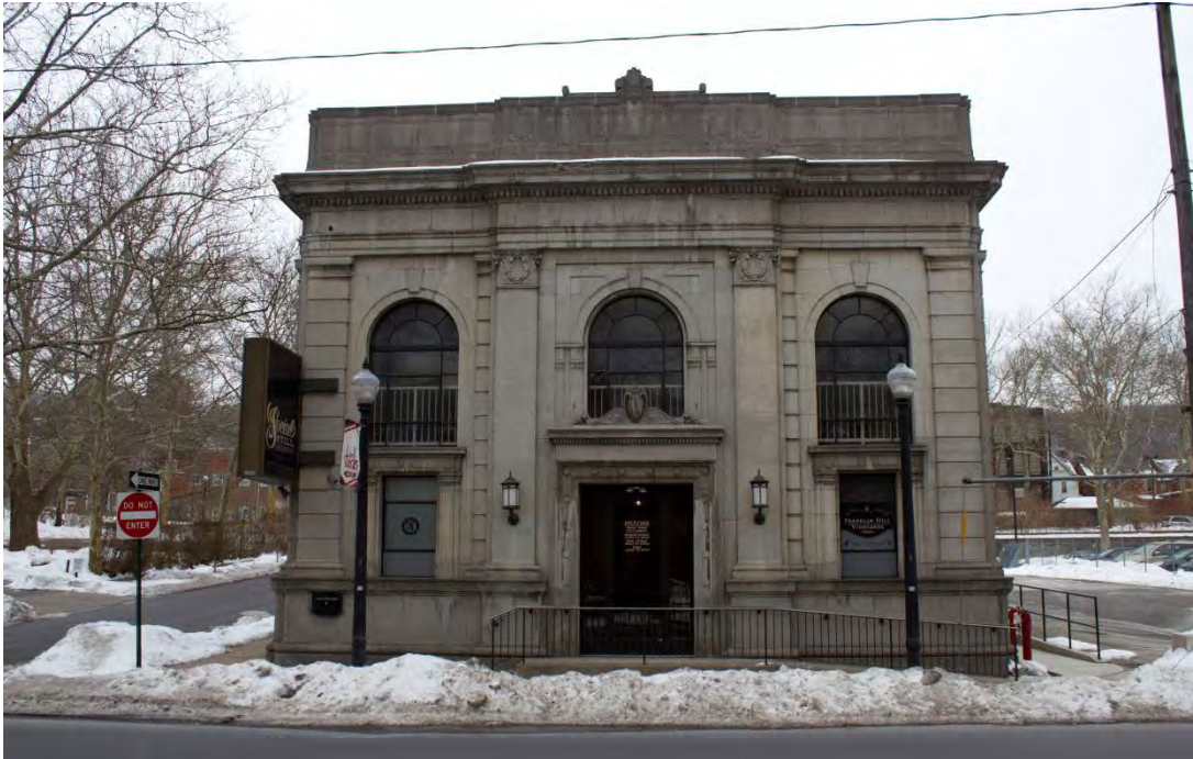
Photo 1—Primary façade from 3 rd Street, facing south.
