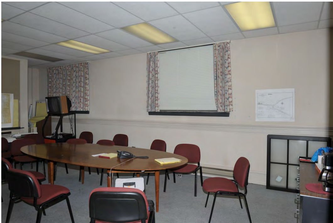
Figure 5: Looking west in the main banking space at the conference room before the removal of the infill and drop ceiling that divided and hid the prominent arched windows, pre-2014 rehabilitation project.
