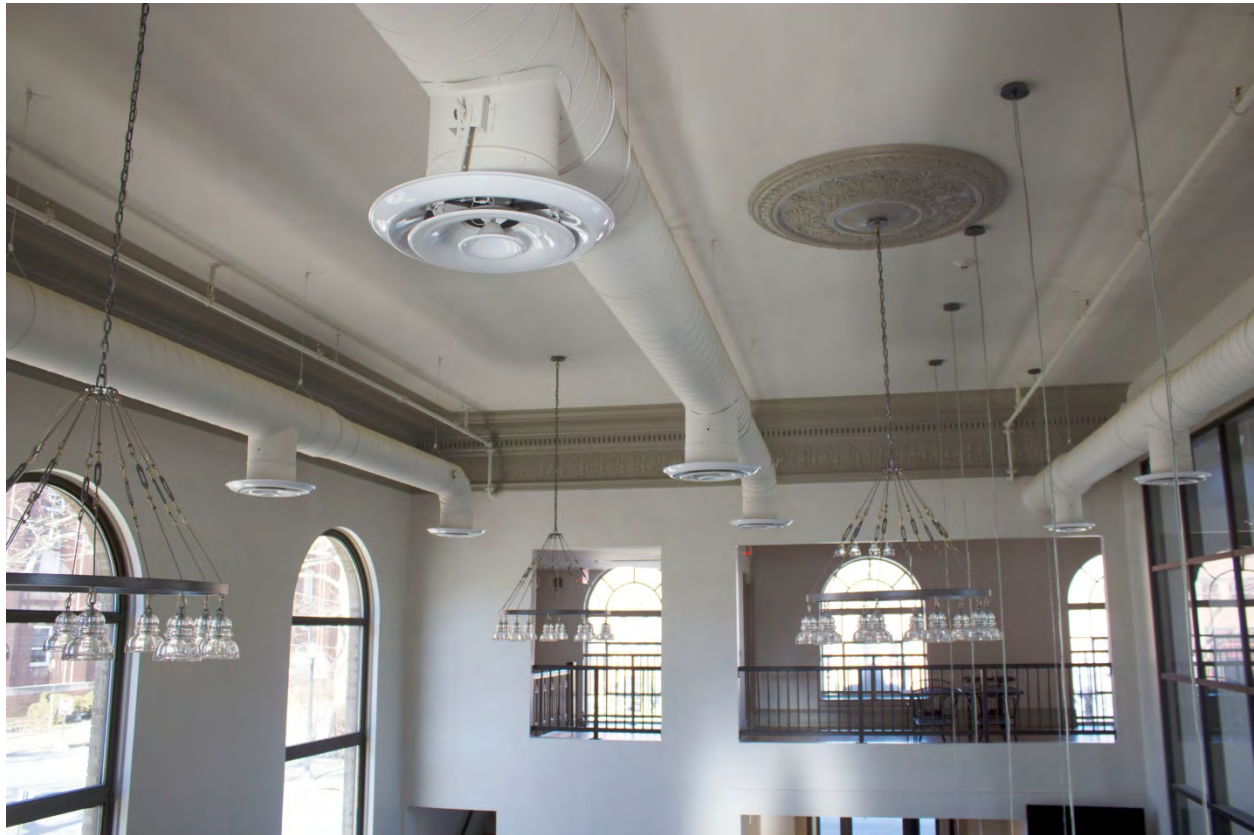
Photo 17—Interior, ceiling detail, showing original medallion and cornice trim, facing N.
