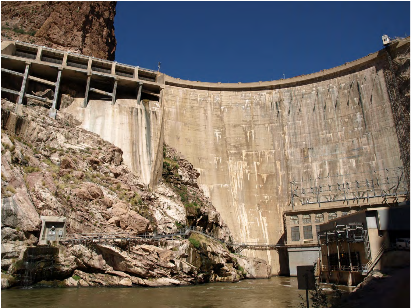
Photo 3: Horse Mesa Dam looking northeast.
