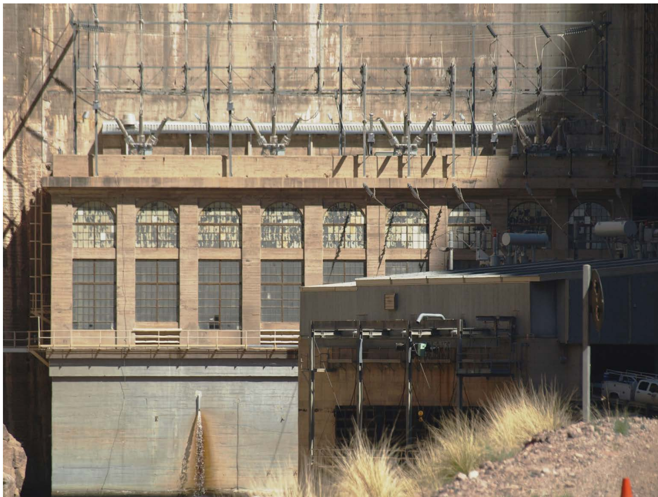
Photo 7: Powerhouse looking east.
