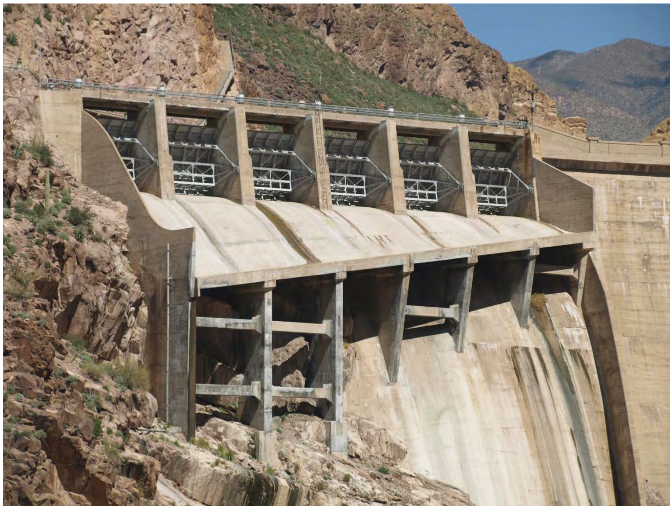
Photo 6: Right spillway looking north.
