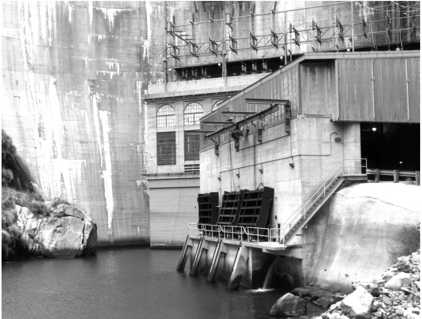
Historic Photo 8. View to the right (west) showing the HEFU turbine unit housing and original power plant of the Horse Mesa Dam. Photo taken in 1988 by Mark Durben. Photo courtesy of the SRP.
