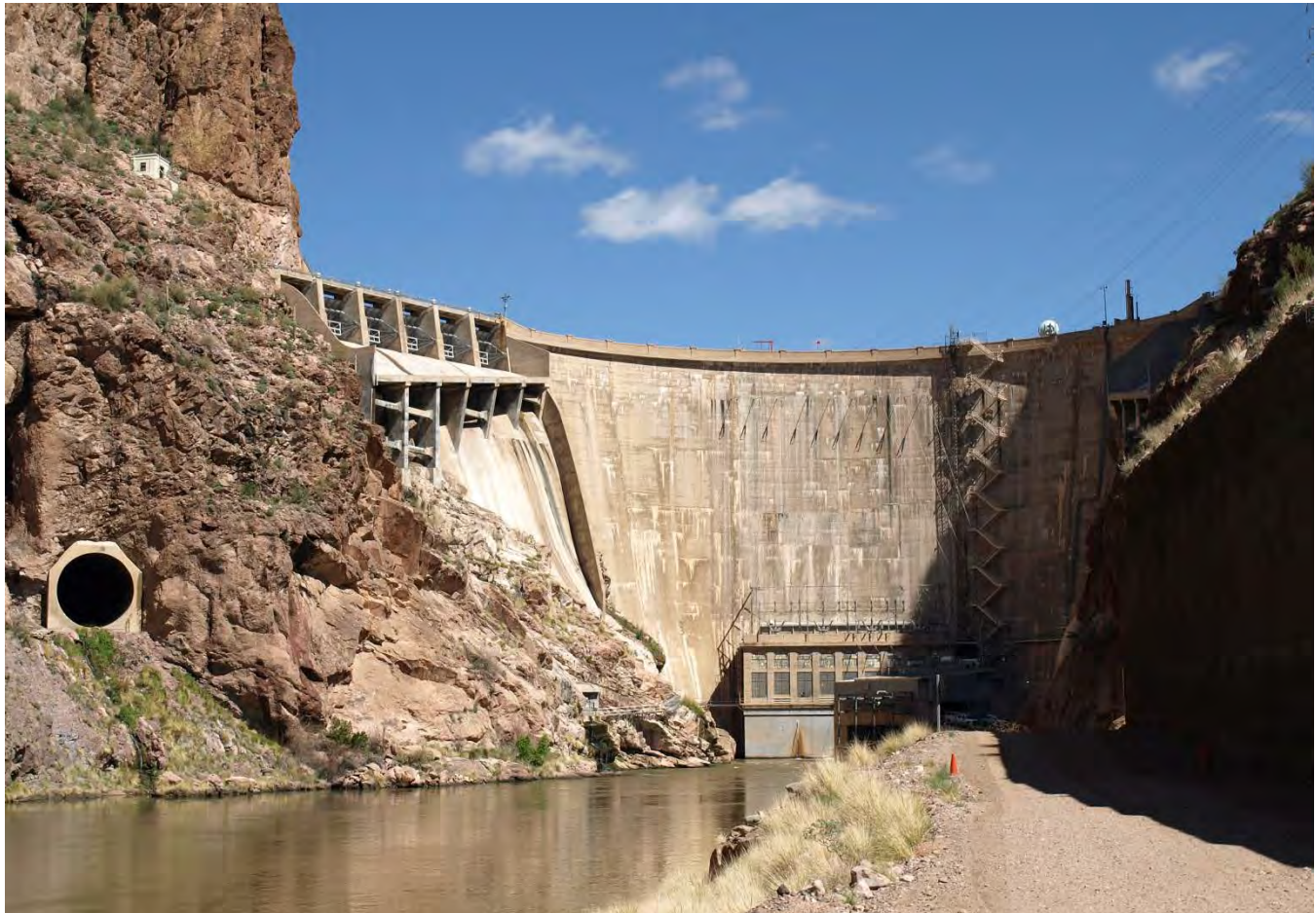
Photo 2: Horse Mesa Dam looking northeast.
