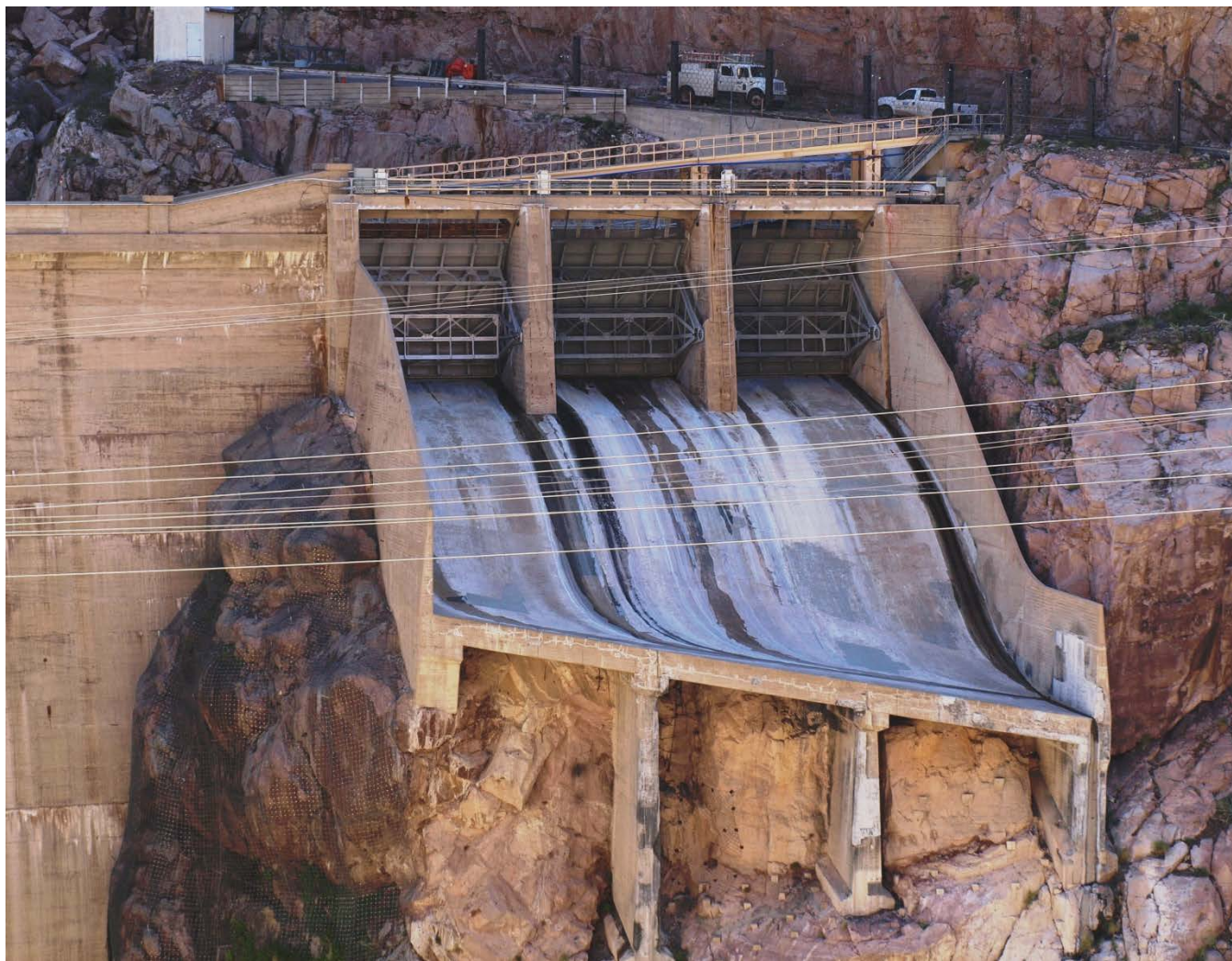
Photo 5: Left spillway from crest looking southeast.
