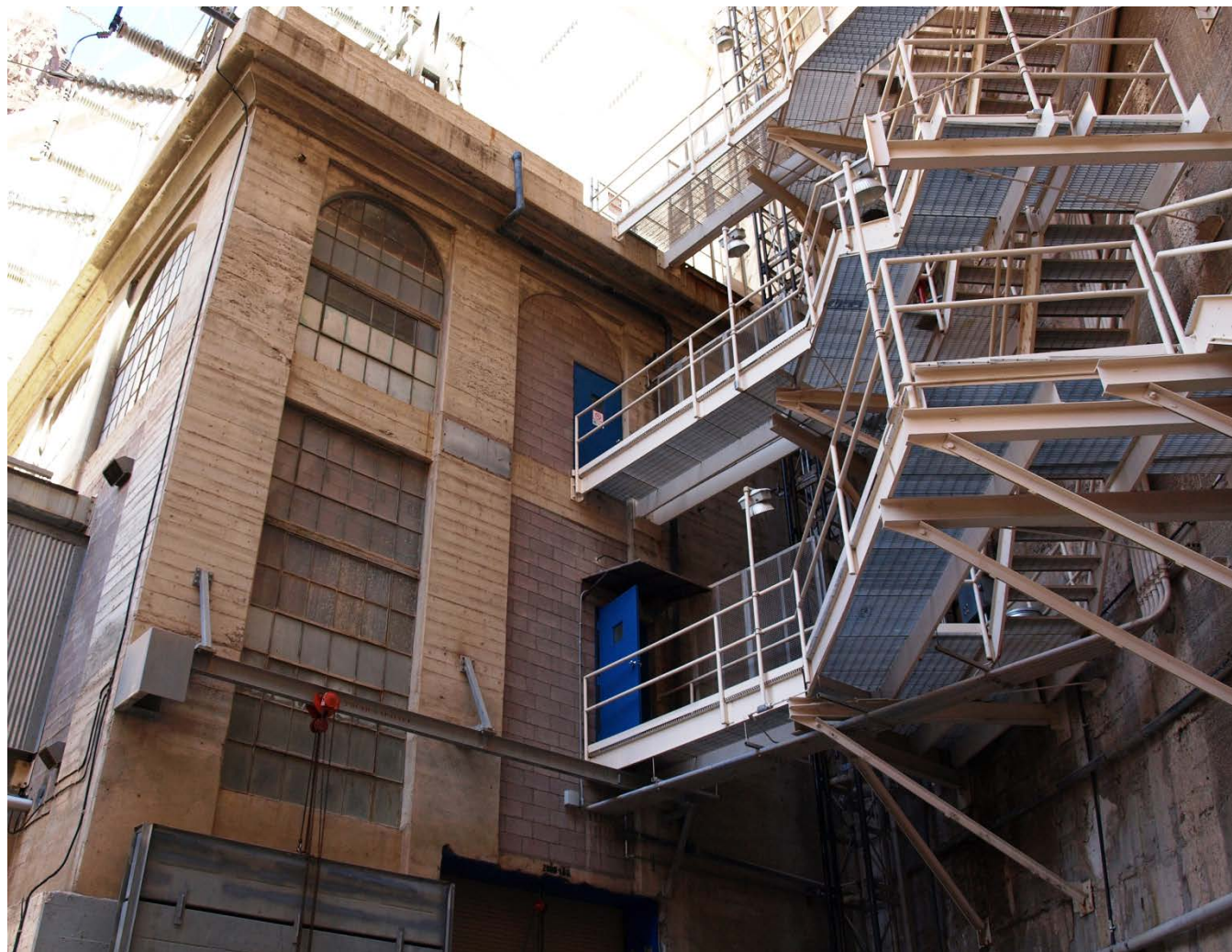
Photo 8: Powerhouse from below.
