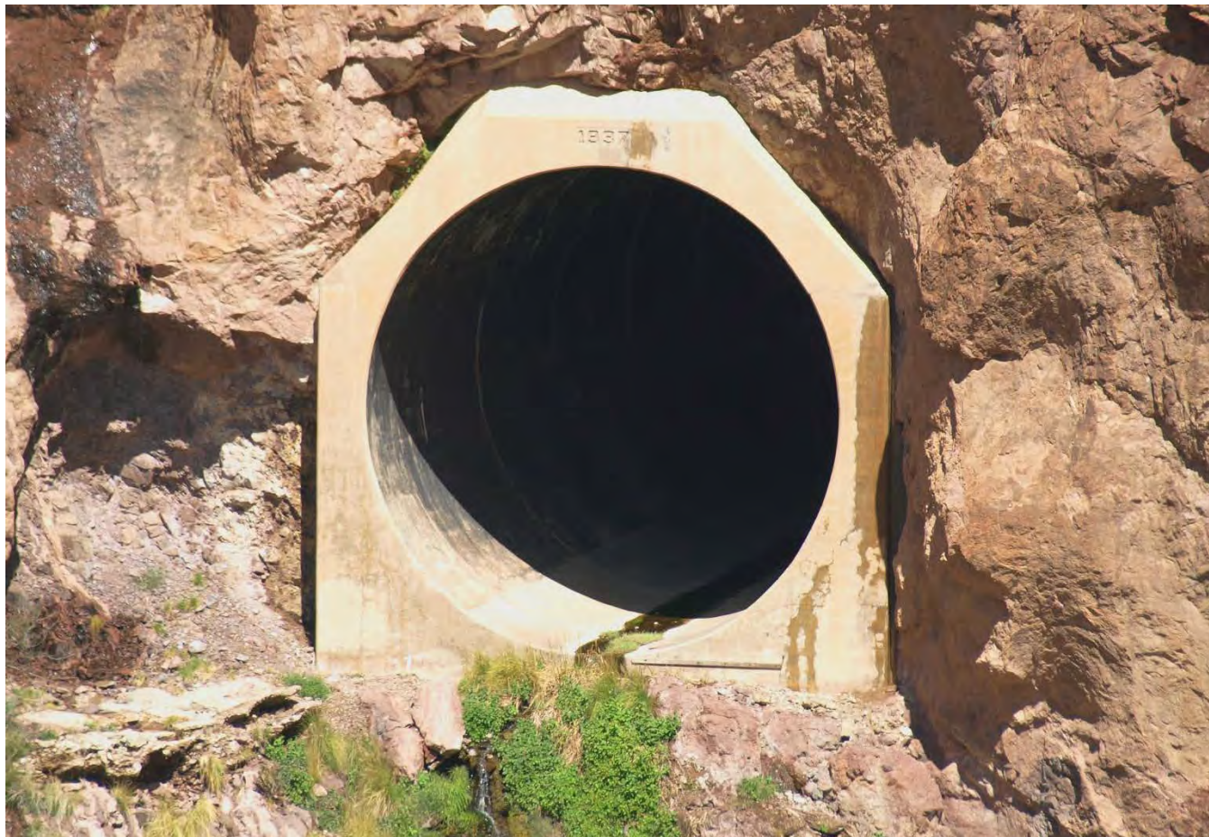
Photo 9: Spillway outlet tunnel looking northeast.
