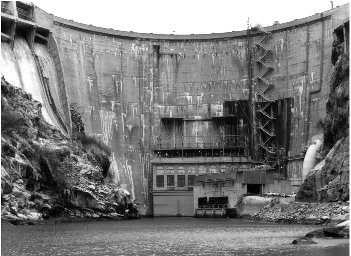
Historic Photo 7. Dam completed except for transformer equipment being installed above the power plant. Photo taken in 1988. Photo courtesy of the SRP.
