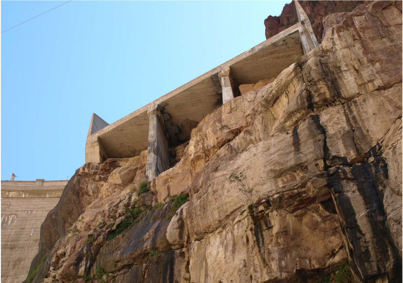
Photo 4: Left spillway looking southeast.
