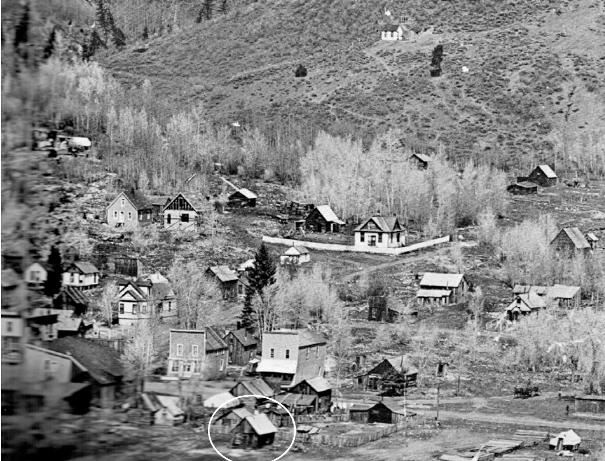
Figure 2. This detail of a ca. 1910 photograph shows the town (with the jailhouse indicated) as taken from the Quarry Road. The jailhouse appears to have a multi-lite window and a metal roof with seams. Photographer unknown; from McCollum, Marble: A Town Built on Dreams , p. 163.
