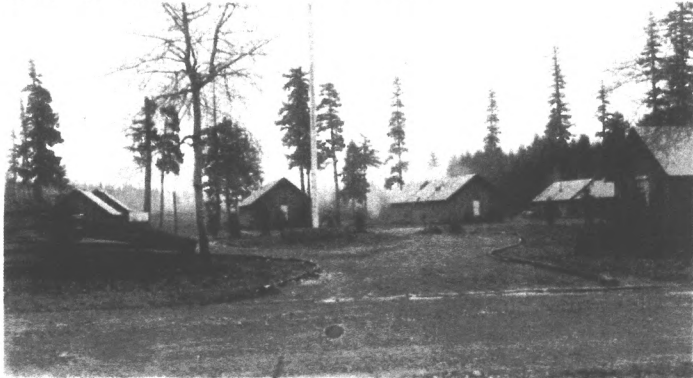
22 Entrance Camp Millersylvania before improvement.
