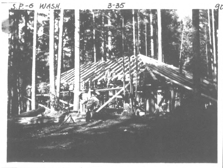
Kitchen #1, framing rafters, March 1935. WSPRC Photo H74.SP-6-90
