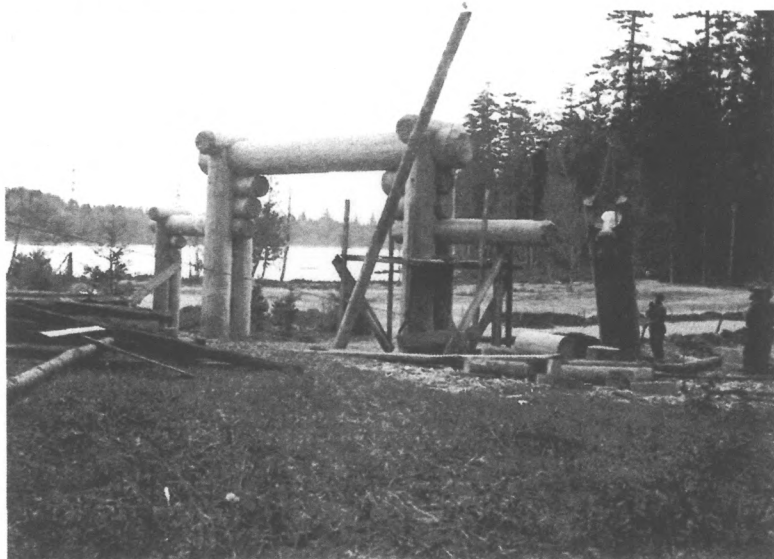
Construction of Park Entrance Sign, May 1935. WSPRC Photo H74.SP-6-119.
