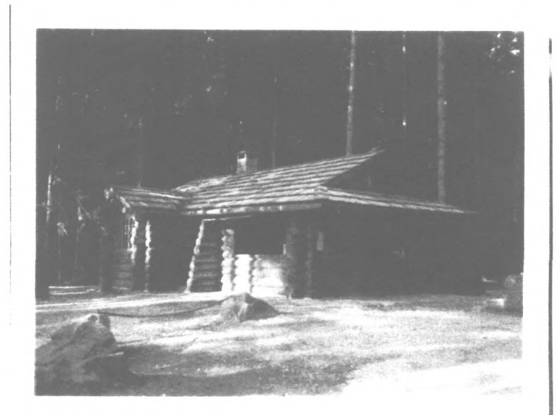
Completed Park House/Concession Stand, n.d. WSPRC Photo H74.SP-6-157
