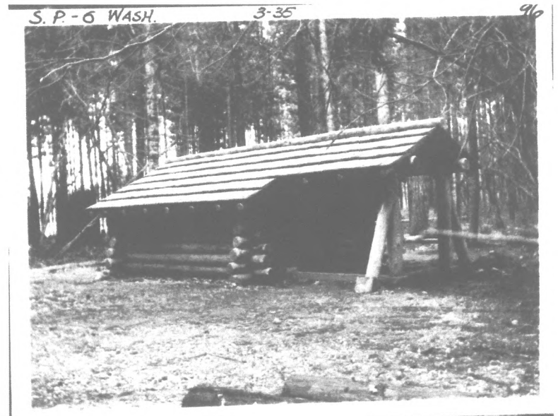
Completed Pump House, March 1935. WSPRC Photo H74.SP-6-96
