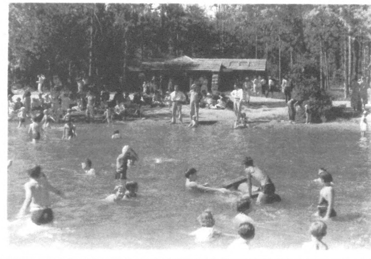
Completed Bathhouse #1, n.d. WSPRC Photo.
