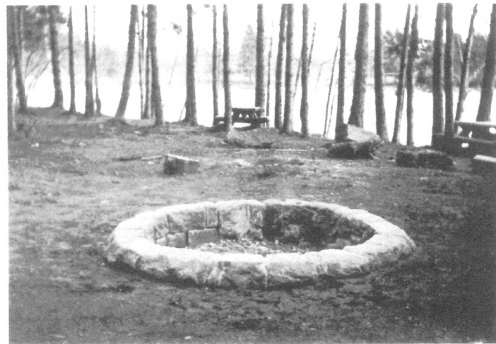
Completed Fire Ring, March 1936. WSPRC Photo H74.SP-6-193
