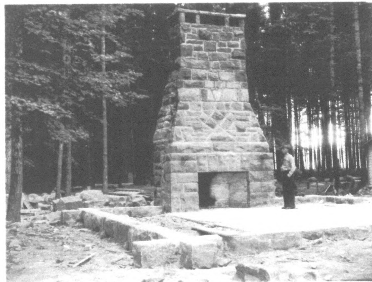
Completed fireplace for Kitchen #2, July 1936. WSPRC Photo H74.SP-6-126
