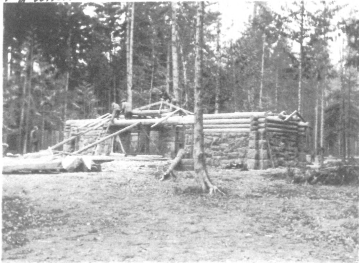
Placing rafters on Bathhouse #2, November 1935. WSPRC Photo H74.SP-6-55
