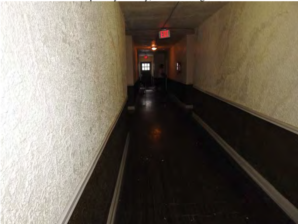
Photo 0008 – First floor primary hallway, camera facing south. Hardwood floors are original.
