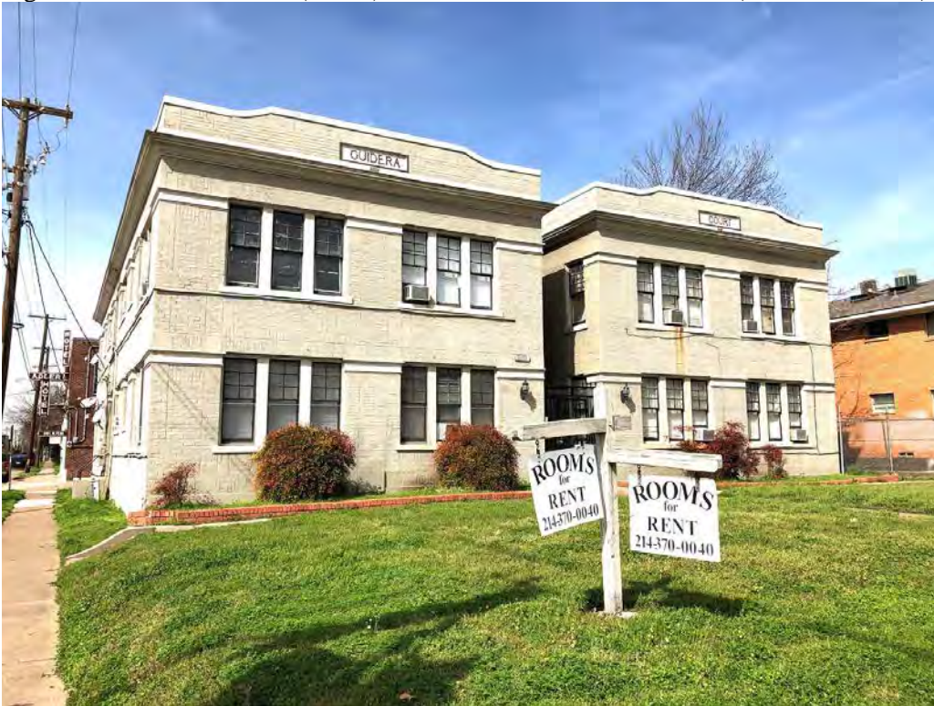
Figure 10 - Guidera Courts (1920c) northeast corner Gaston at Peak (Architexas 2019)
