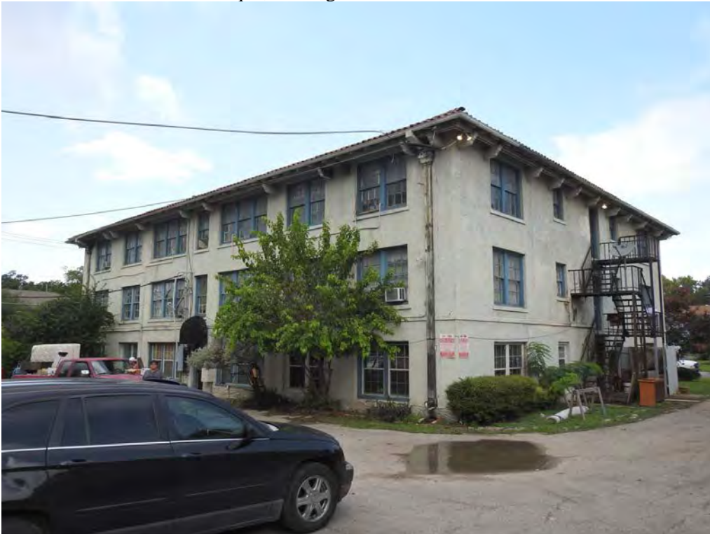
Photo 0004 – Southeast oblique, looking northwest.
