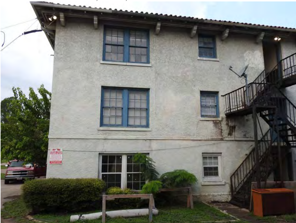
Photo 0005 – East elevation, cornice, and window detail.
