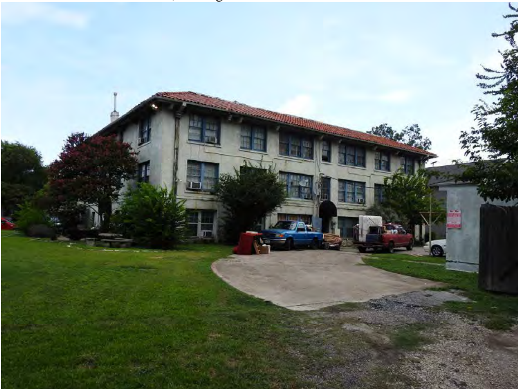
Photo 0003 – South elevation, looking northeast.
