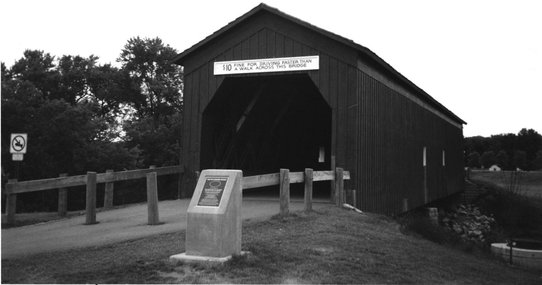
Zumbrota Covered Bridge Goodhue Co., MN 013380 - 0/0A
