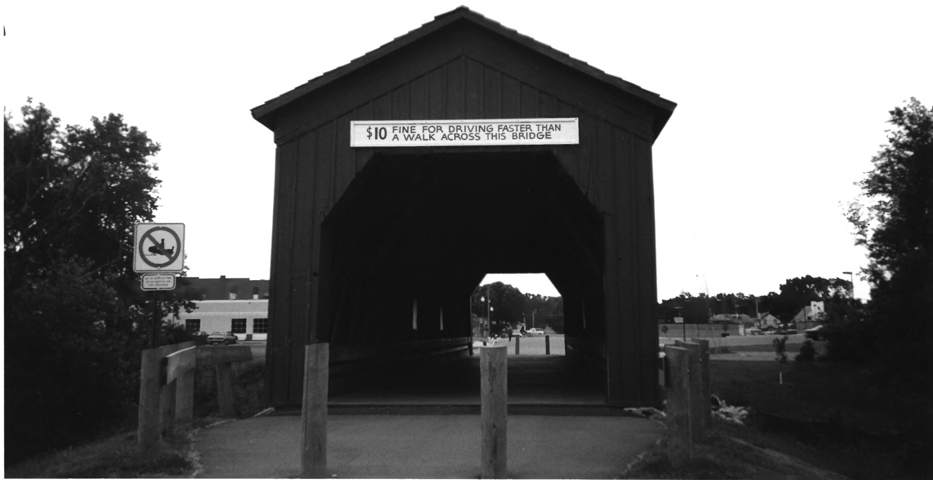
Zumbrota Covered Bridge Goodhue Co., Mn 013380-4/4A
