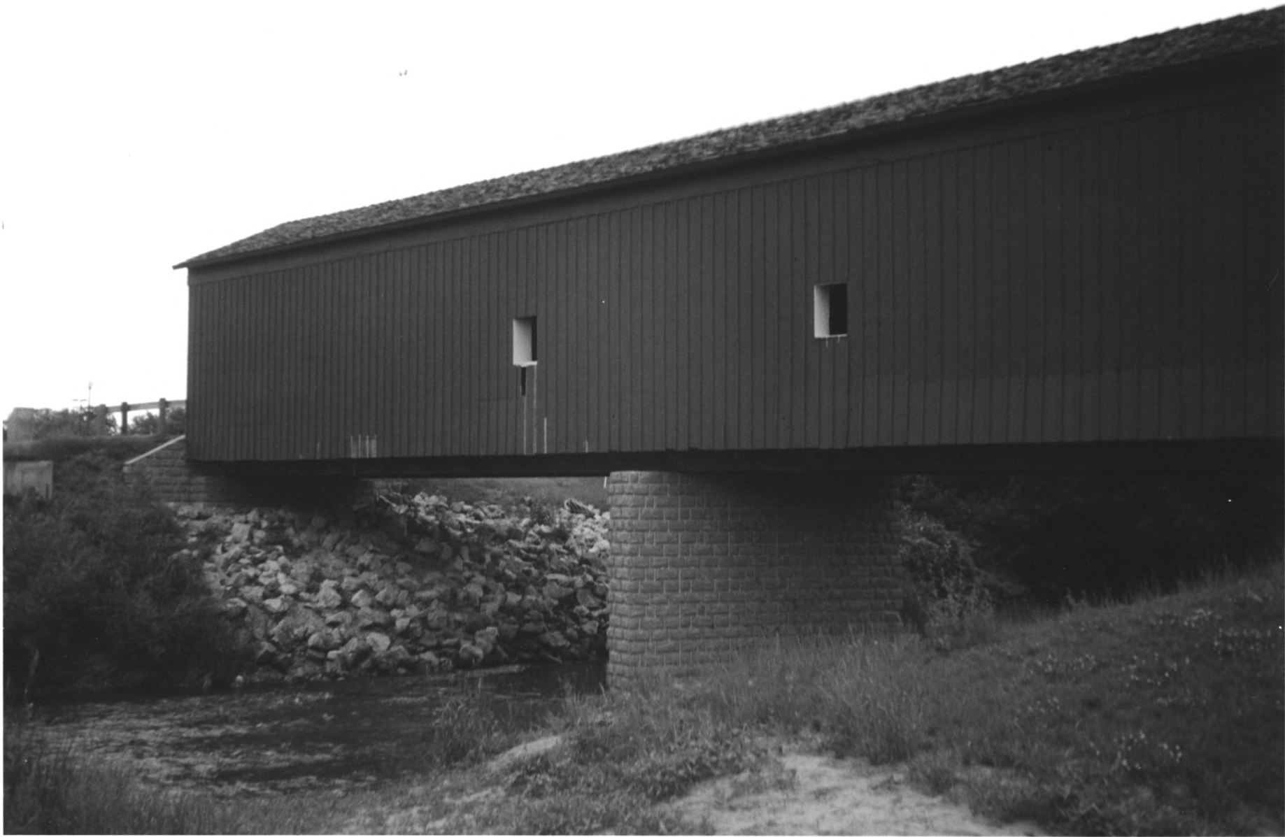
Zumbrota Covered Bridge Goodhue Co., Mn 013380-8/8A
