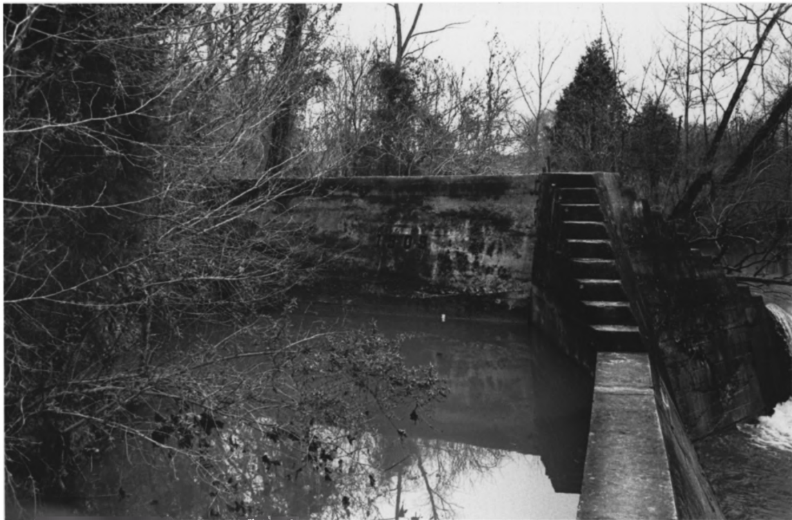
Sparta Hydroelectric Station Sparta vicinity, White County, TN
