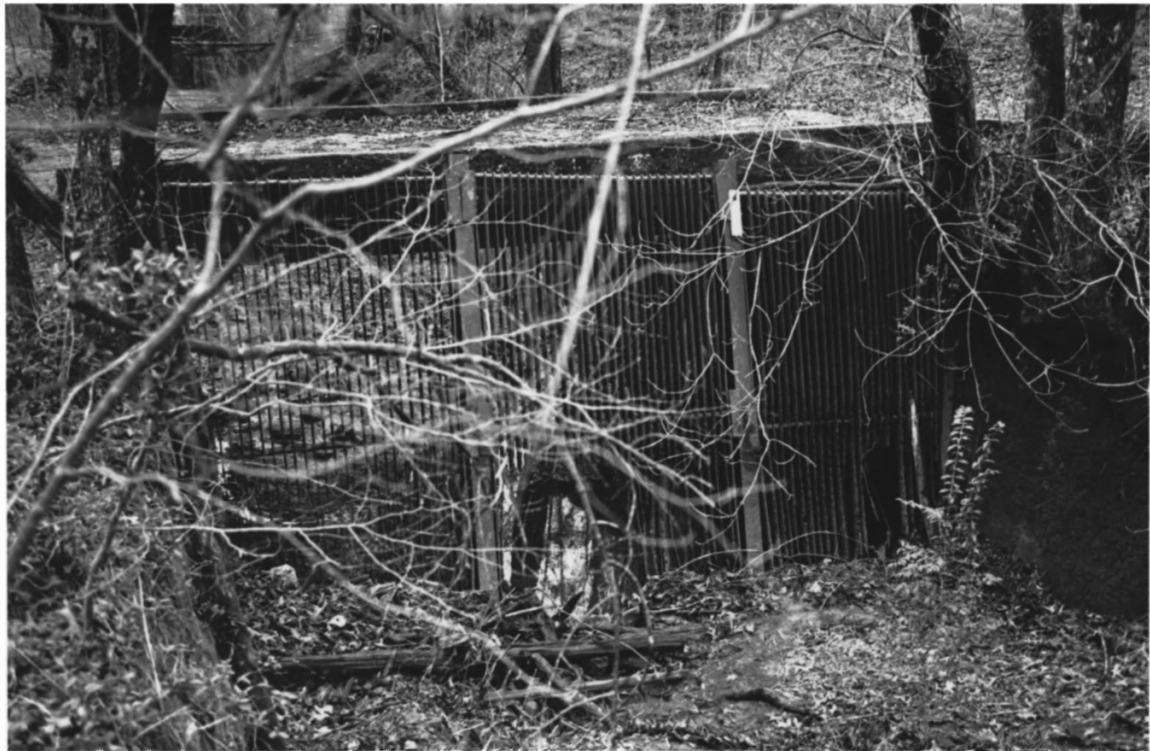
Sparta Hydroelectric Station Sparta vicinity, White County, TN
