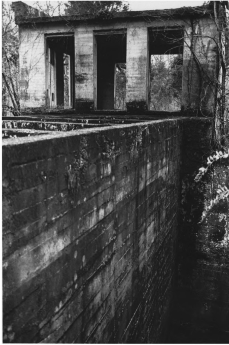
Sparta Hydroelectric Station Sparta vicinity, White County, TN
