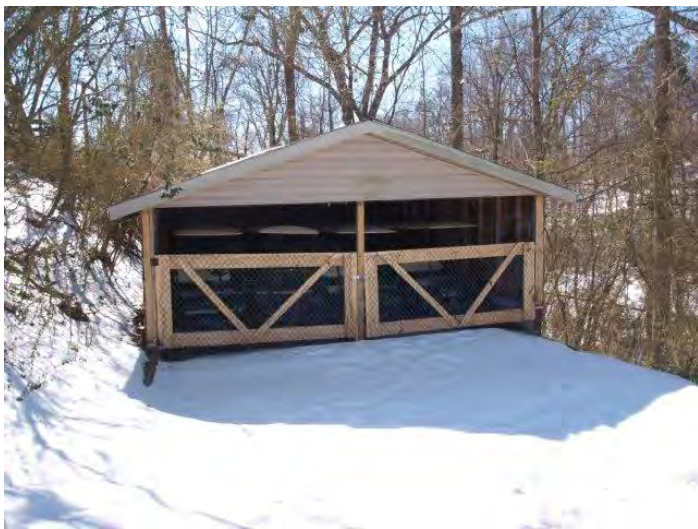
Cart House (photo 15)
