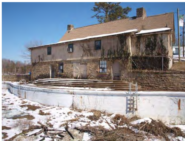
Photo 13: West side (back)
