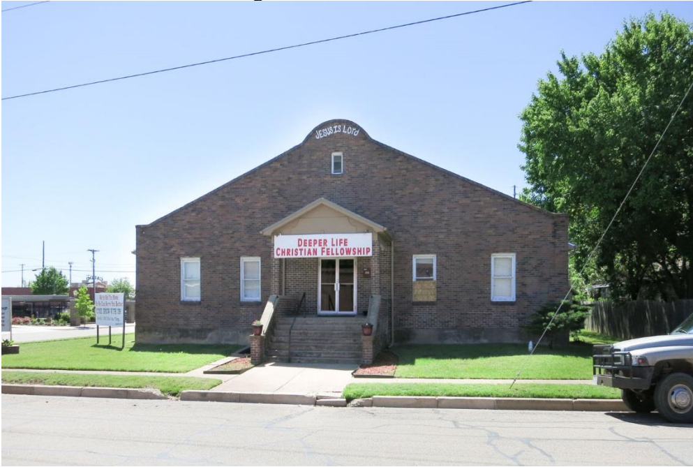
Photo 45 Building at 104 S. Robinson Street (Property #122) East elevation, camera facing west
