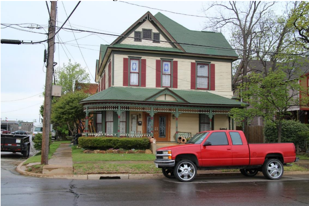
Building at 201 N. Anglin Street (Property #2) East elevation, camera facing west
