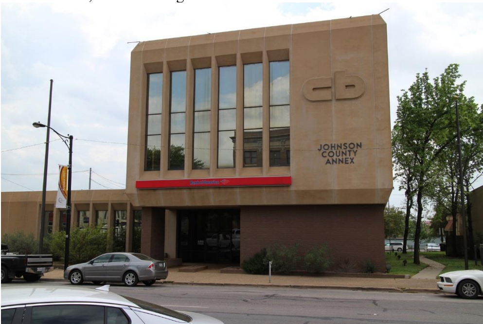
Photo 48 Building at 1 N. Main Street (Property #84) – Noncontributing / Outside Period of Significance East elevation, camera facing west
