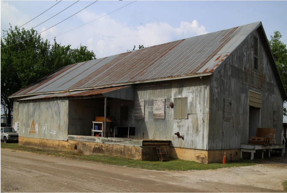
Photo 17 Building at 102 S. Border Street (Property #8) Northeast oblique, camera facing southwest
