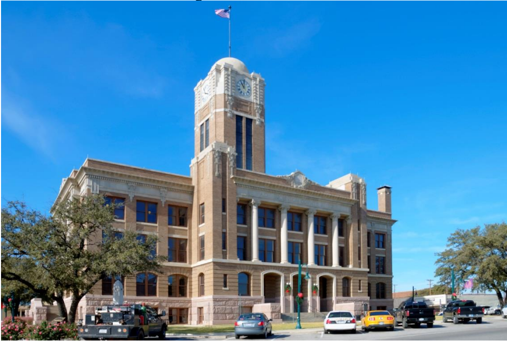
Photo 47 Johnson County Courthouse (Property #85) South elevation, camera facing northeast
