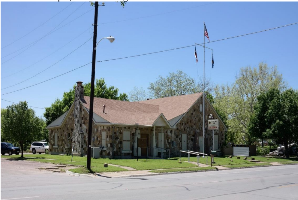
Photo 28 Building at 313 W. Chambers Street (Property #52) Northeast oblique, camera facing southwest
