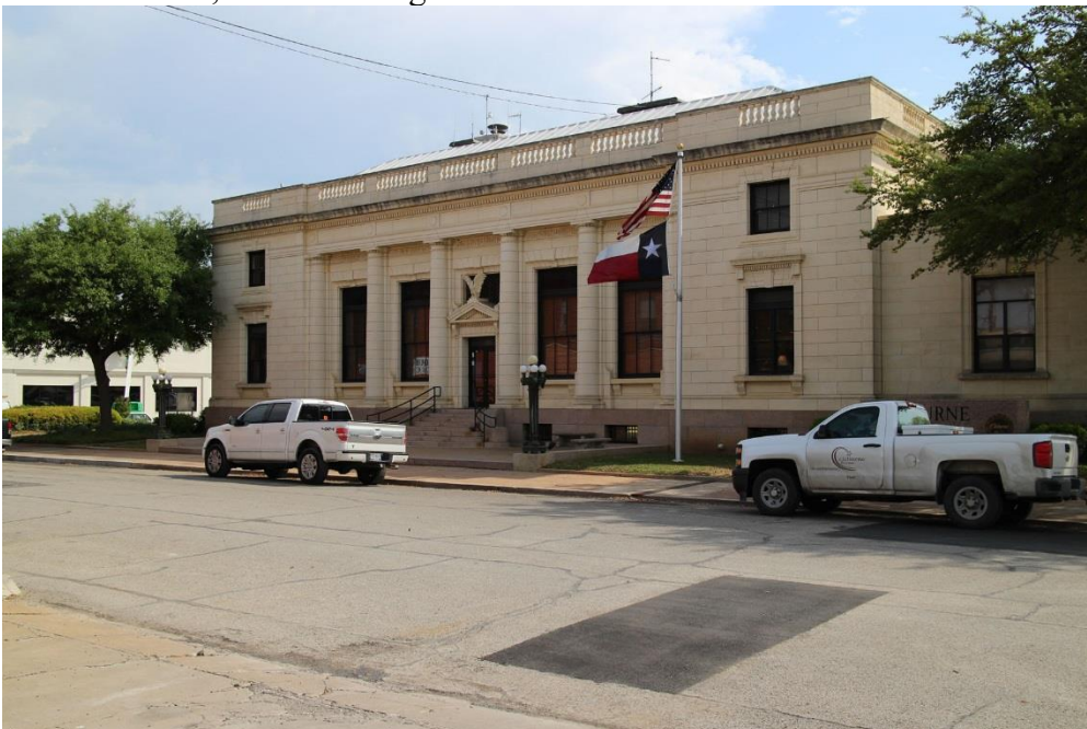
Photo 44 Building at 10 N. Robinson Street (Property #119) West elevation, camera facing northeast
