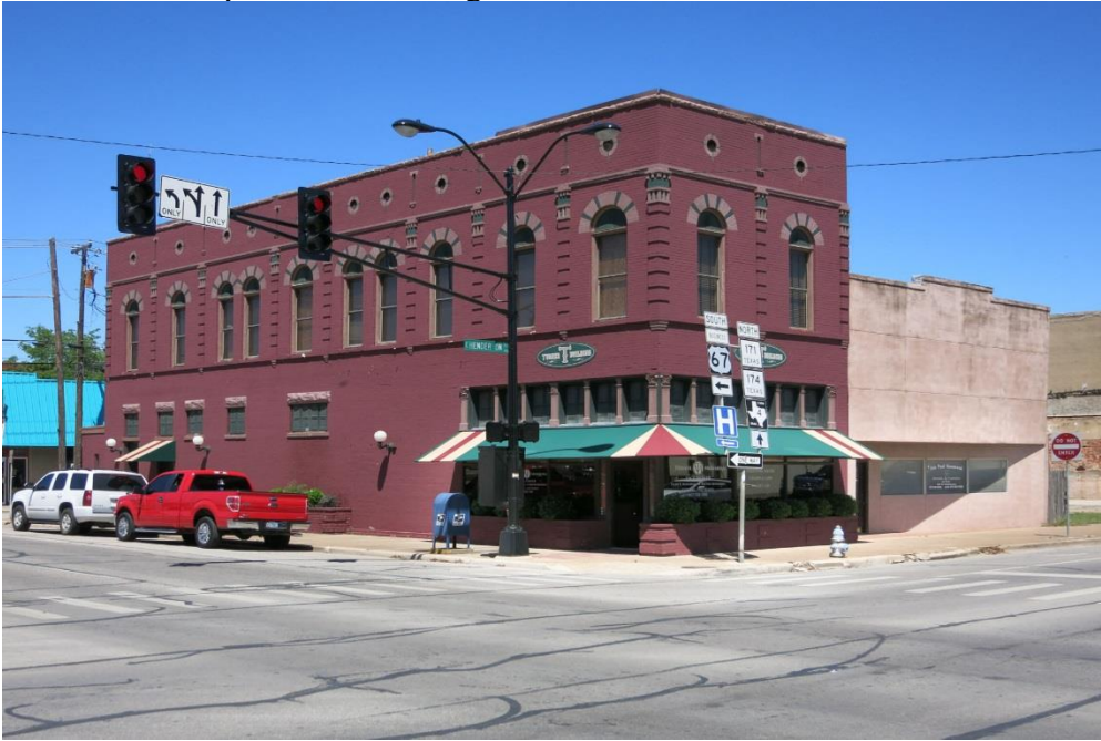
Photo 29 Building at 101 E. Henderson Street (Property #57) Southwest oblique, camera facing northeast
