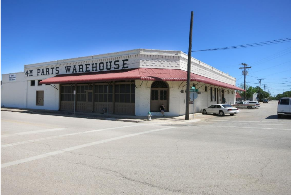
Photo 27 Building at 402 E. Chambers Street (Property #48) Northwest oblique, camera facing southeast
