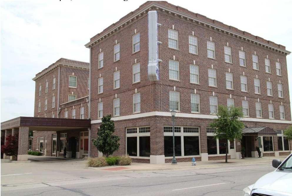
Photo 23 Building at 205 S. Caddo (Property #24) Northwest oblique, camera facing southeast
