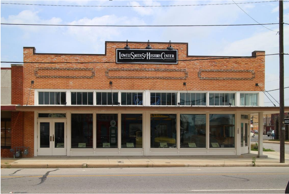
Photo 37 Building at 200 N. Main Street (Property #91) West elevation, camera facing east
