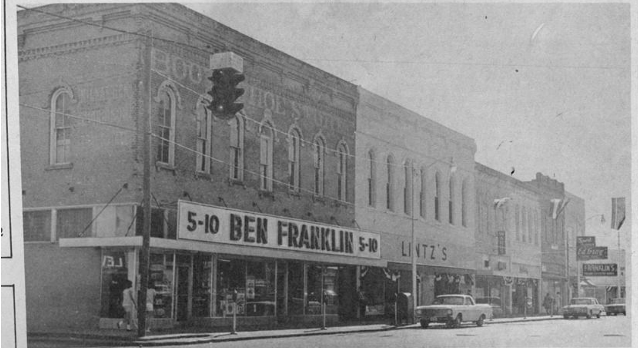
South Side of Square 1967
