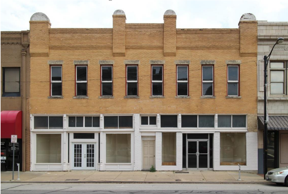
Photo 19 Building at 6-8 N. Caddo Street (Property #10) West elevation, camera facing east
