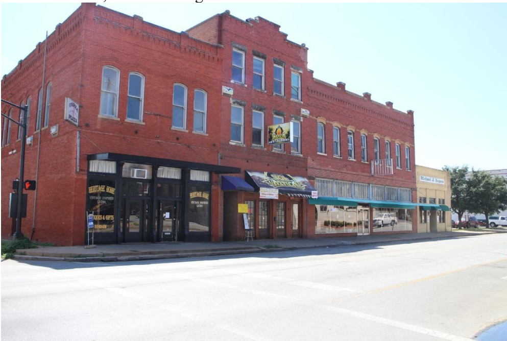
Photo 10 Buildings at 108 through 114 E. Chambers Street North elevation, camera facing southwest
