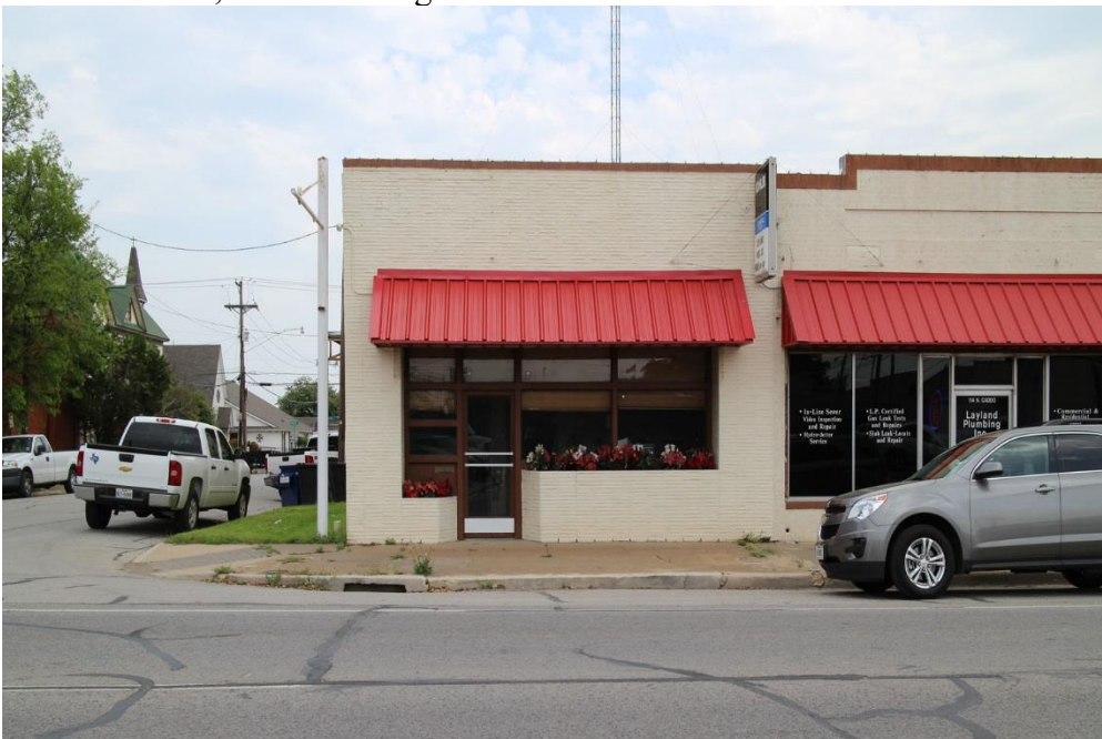
Photo 20 Building at 116 N. Caddo Street (Property #16) West elevation, camera facing east
