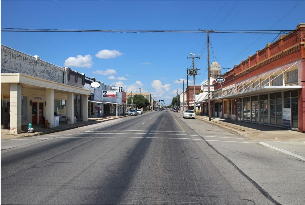
Photo 5 Streetscape of S. Main Street Camera facing north along S. Main Street at W. Harrell Street
