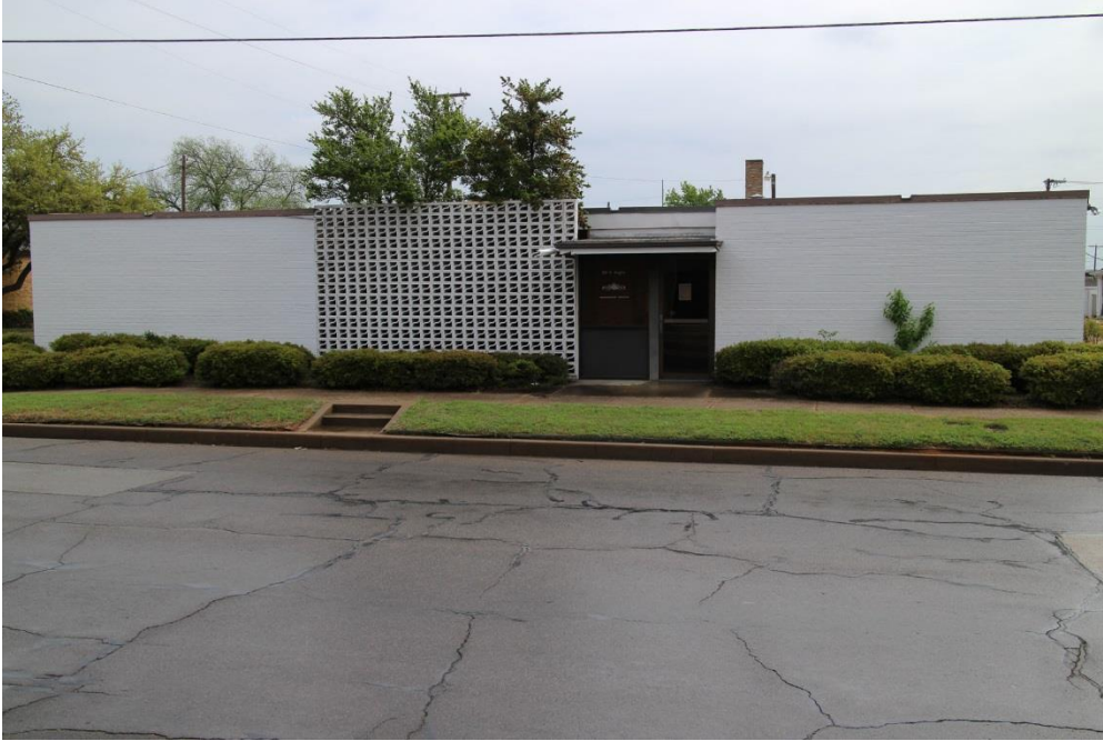
Photo 15 Building at 212 N. Anglin Street (Property #5) West elevation, camera facing east
