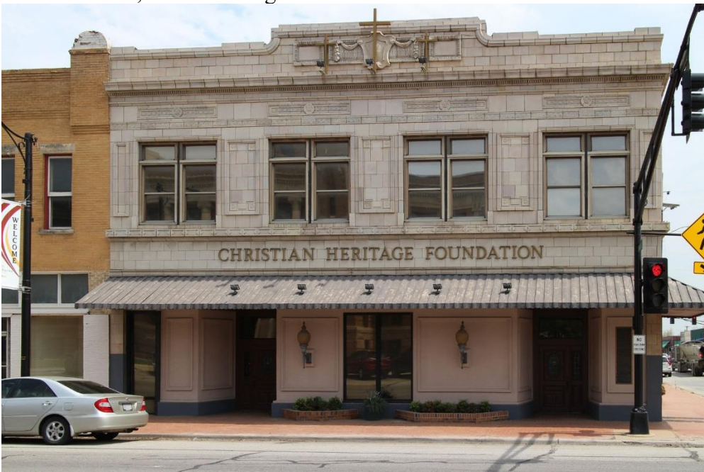
Photo 18 Building at 2-4 N. Caddo Street (Property #9) West elevation, camera facing east
