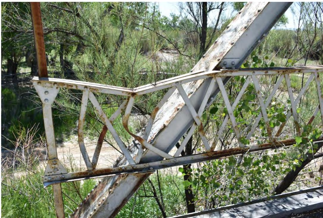
15 of 15. Lattice railing damage detail. Camera facing southeast.
