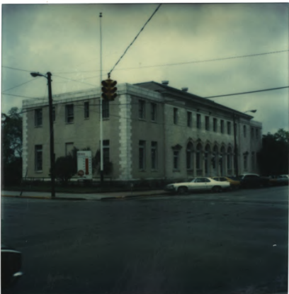
FRONT OF BUILDING 605 ELIZABETH STREET
