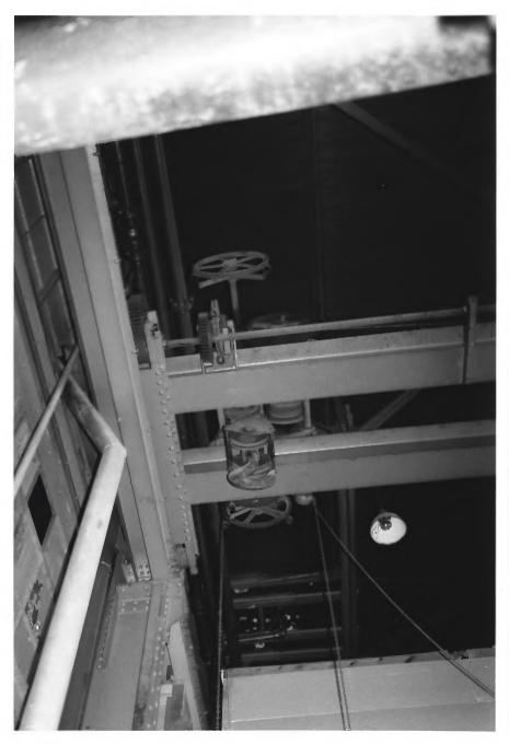
Detail of overhead hoist and steel track for working on diesel generators.
