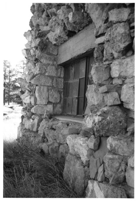
Corner of power house showing stone and concrete work and steel-sash industrial windows. Grand Canyon Power House
